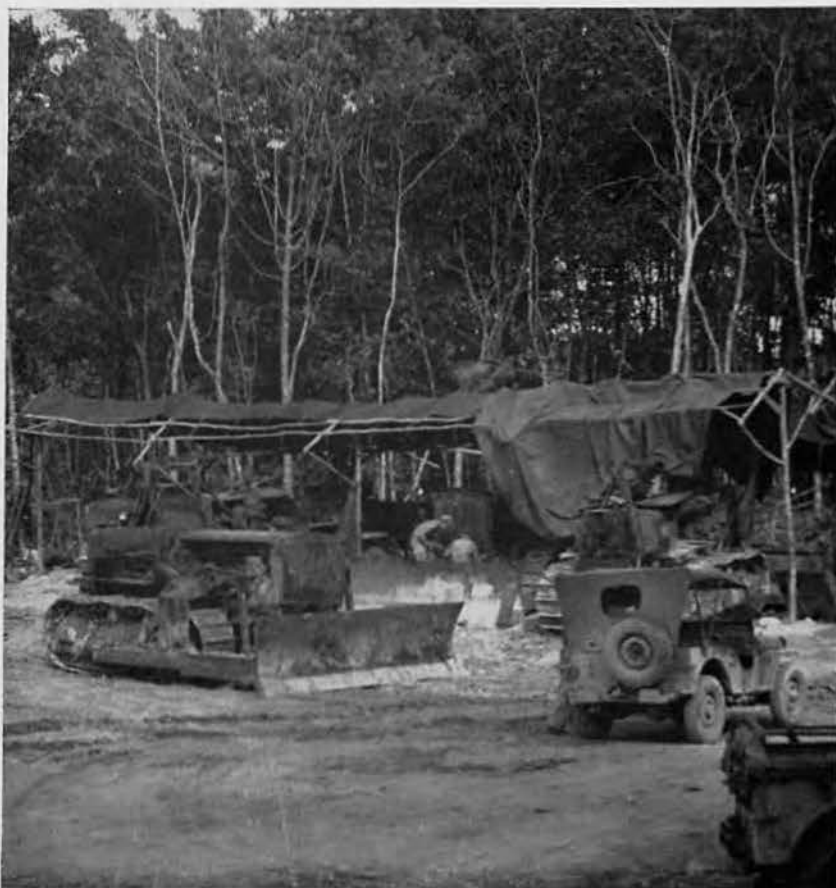
BIG STUFF. Vital to the sustained construction progress of Stirling Field was the essential work done by the highly skilled crew of the Heavy-Duty Machine Shop on such monstrous earthmoving equipment as power shovels, carryalls, bulldozers and motor graders.
