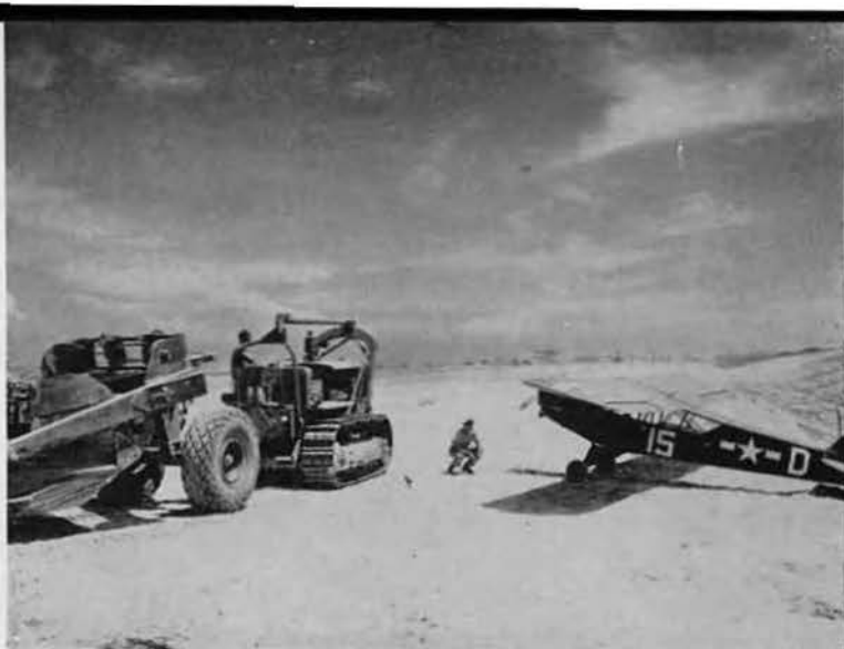
STINSON GRASSHOPPERS were first planes to use Bolo Field. During very first week of construction 'Hoppers landed and took off on west shoulder of strip. Clyde Pemberton inspects mite from his 'dozer as Chief Ken Hansing crouches.
