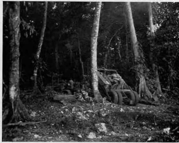
MORE PROVISIONS ARRIVE. A monstrous carryall, jampacked with vitally-needed supplies and provisions for early occupation forces on Stirling, rumbles cautiously down a tortuous road, blazed only a few hours earlier by a sweating Seabee and his bulldozer.
