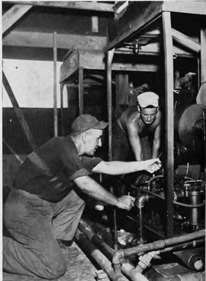
BOILER CHECK. Mike Yanoscik (left) and Martin Melasky check valves of boilers supplying hot water and steam for sterilizing operation. Despite most modern methods of design, this plant, built in July, was destroyed by terrible typhoon of 9 October.
