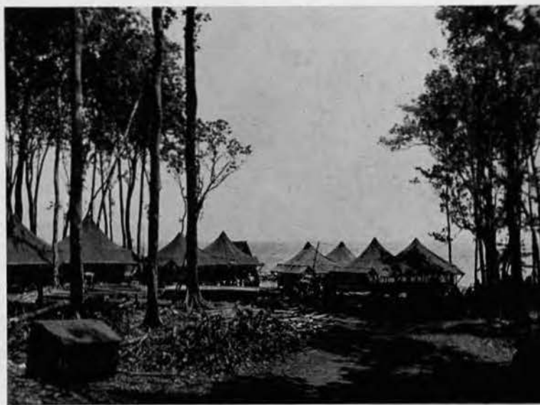
PILOTS CAMP is well under construction. Carpenters (center) are completing tent decks. Replete with screening and framework, these tents provided cool, comfortable living quarters for combat-weary P-38 pilots at Stirling. A mess hall and shower rounded out camp.
