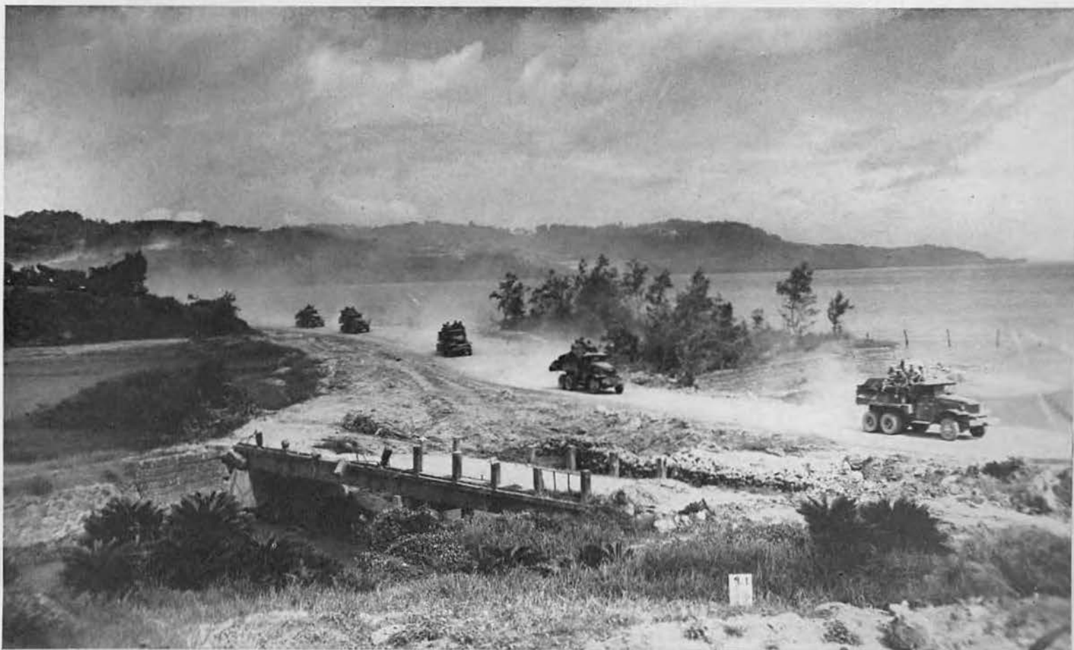
BATTLE-WEARY VETERANS are speeded back from front lines over Route 6, which 87th Earthmovers converted from a jeep trail to a main thoroughfare. The project was under the supervision of Lt. Toivo Panttaja. This
