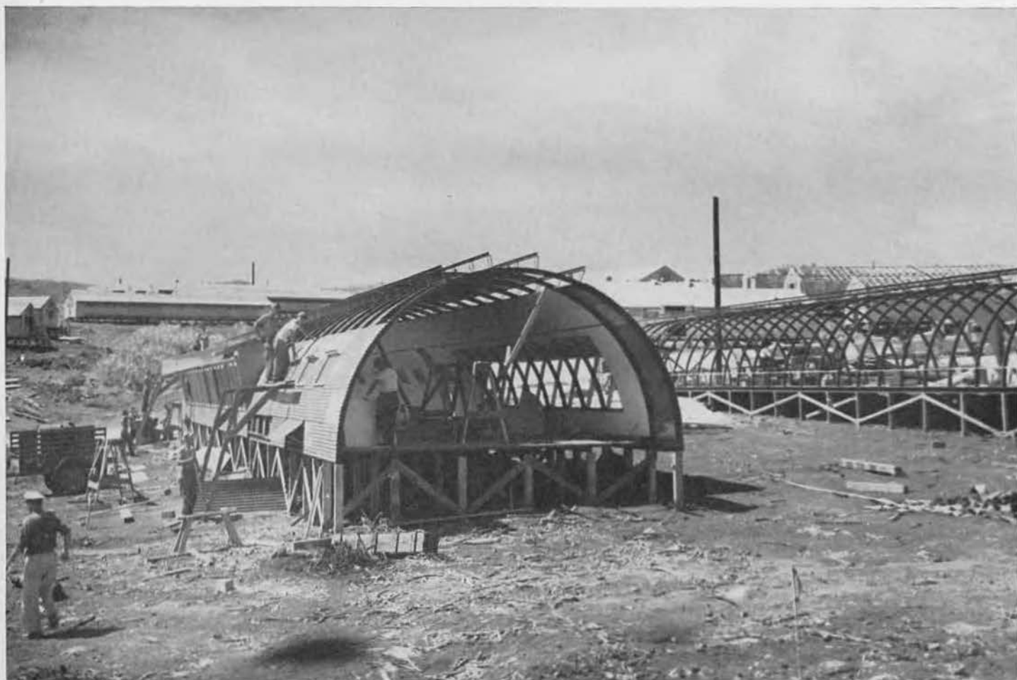
39TH GENERAL HOSPITAL was one of three projects assigned the 87th during its three-month stay on Saipan. Above quonset hut additions provided cool, roomy wards for wounded Marines returning from the flaming inferno that was Iwo Jima in February. This hospital assignment was, in
