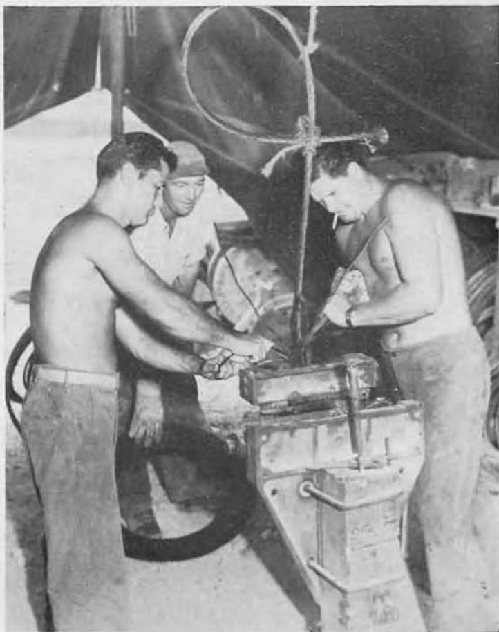
TRANSPORTATION RIGGING LOFT. The cable crib was no place for gold-bricks. Here, T Division riggers took care of cables for shovels, cranes, draglines, etc. Chief Charlie Bowers (center) assists as Tom Nanfra (left) holds strands and Joe Basket applies spike.
