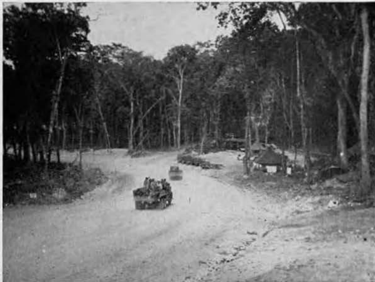
A MAIN DRAG on Stirling Island—a section of beach highway approaching the entrance road to ACORN 12 and the Pilots Camp area. This super-speedway, originally a trail 'dozed out' by invasion forces, was 40 feet in overall width.
