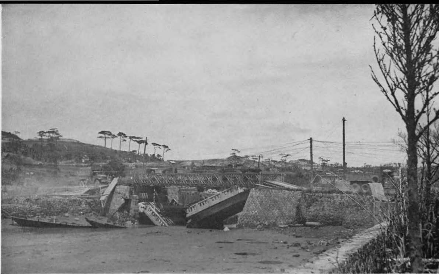
UNBEATABLE. Japs retreating south from Naha to take up final positions blew up this concrete bridge to hamper the American drive. The unbeatable Army Engineers reduced lost time to a minimum by throwing a prefabricated Bailey bridge over the chasm in record time. It was imperative
