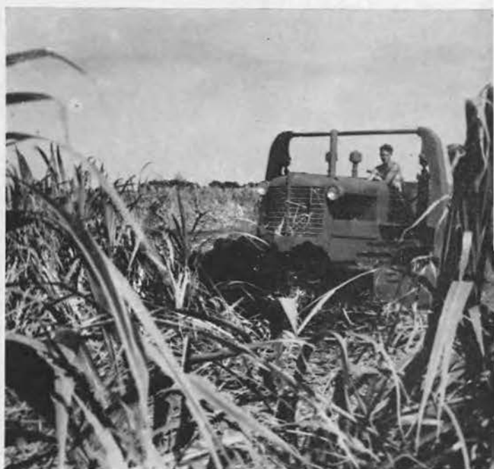
CULTIVATOR. A chugging 'dozer, operated by "Red" Moorman, clears a patch of native sugar cane as camp construction begins in earnest. During the months an entire army was being assembled for the BIVE assault, the 87th sweated it out here.
