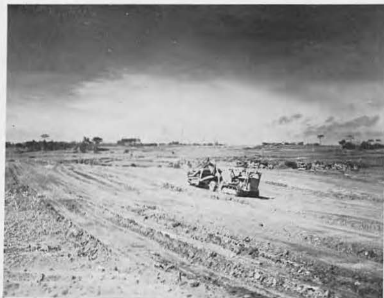
HARVESTING. Widespread vegetation, consisting principally of sweet potatoes and beans, is removed from sub-grade site by pans as 87th assembles maximum skill and power for all-out assault on what is to be its last wartime project.
