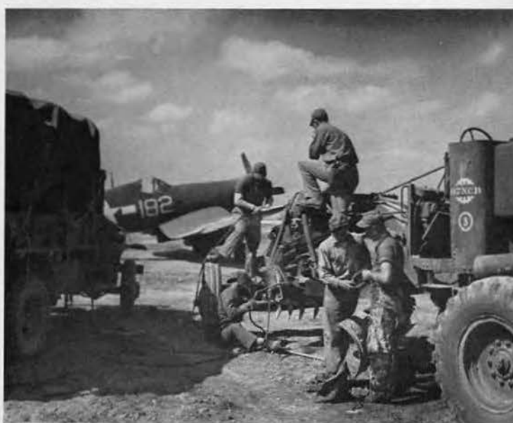
FIELD REPAIRS. Sam Newman (atop his grader) watches "Porky" Clements weld the under parts of his damaged machine. Frank Hevey and Clarence Dean (right), heavy duty mechanics, scrutinize a defective part. Truck (left) contains complete welding equipment.
