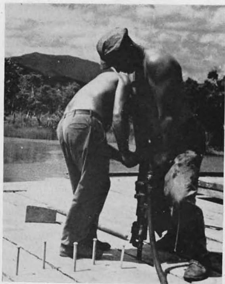
TIE HER DOWN RIGHT THERE! An almost miraculous time-saver was the air-hammer, which practically eliminated the back-breaking sledge hammer and an extra crew. Here, the Jones boys add their combined weight and brawn to vibrating spike-driver.
