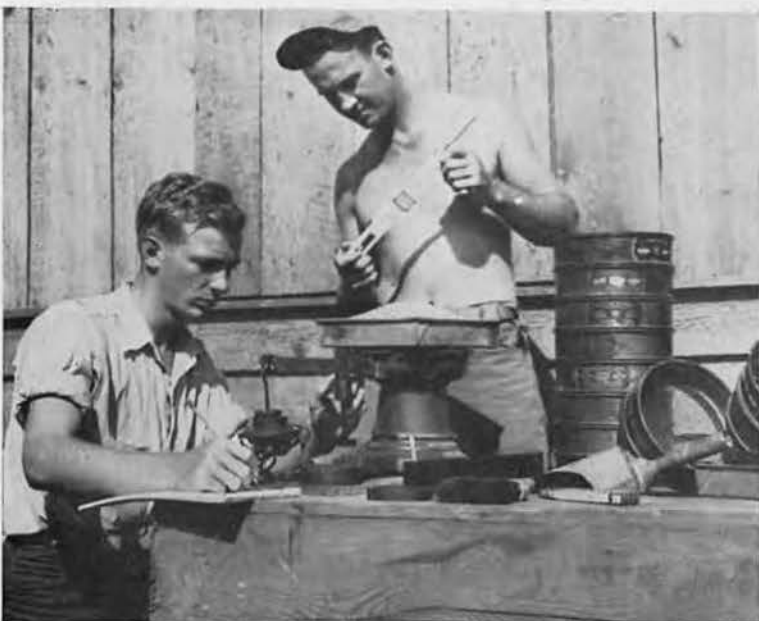
TESTING screened limestone taken at random from storage bins, Ralph Ackerman (left) and Byron Chronic use a slide rule in making computations. Aggregate was thoroughly tested every eight hours to insure minimum specifications.
