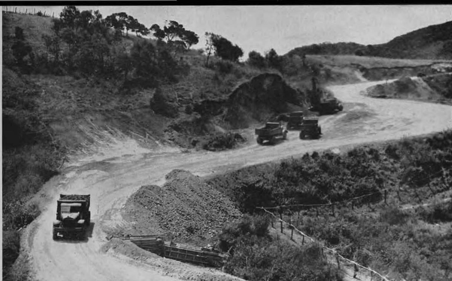
LITTLE BURMA ROAD. Snaking over exceedingly treacherous mountain passes, the original road above Bourail was actually no more than a narrow 15-foot wagon trail. Earth, cut away from the bordering red-dirt bluffs, was dumped over edge on opposite side
