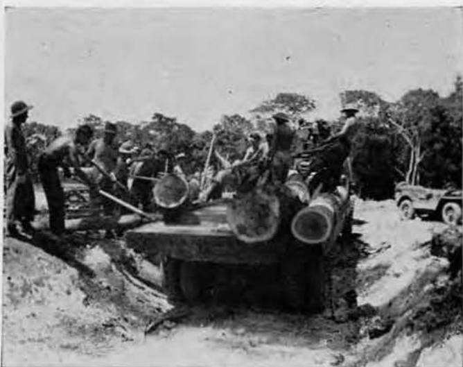
AND THEY CARRIED THEM AWAY TO THE MILL. Lumber for pilot housing was sawed from timber cleared from the Strip. Here, Bos'n's Mate Meredith Walls and crew load out a few. A 'dozer ditch accommodates the trucks and eliminates uphill pull.
