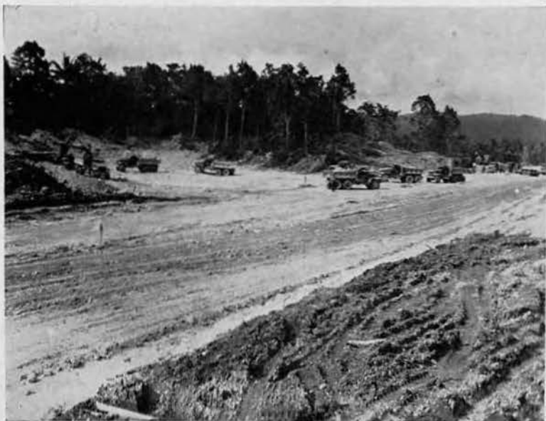
MAKE ROOM FOR BOMBERS! Fighters were already hitting Rabaul from the 5,000-foot completed strip. To make room for bombers, the men turned to taxiways and hardstands. (This 87th photo—one of eight—appears on Page LXII of CAN DO.)
