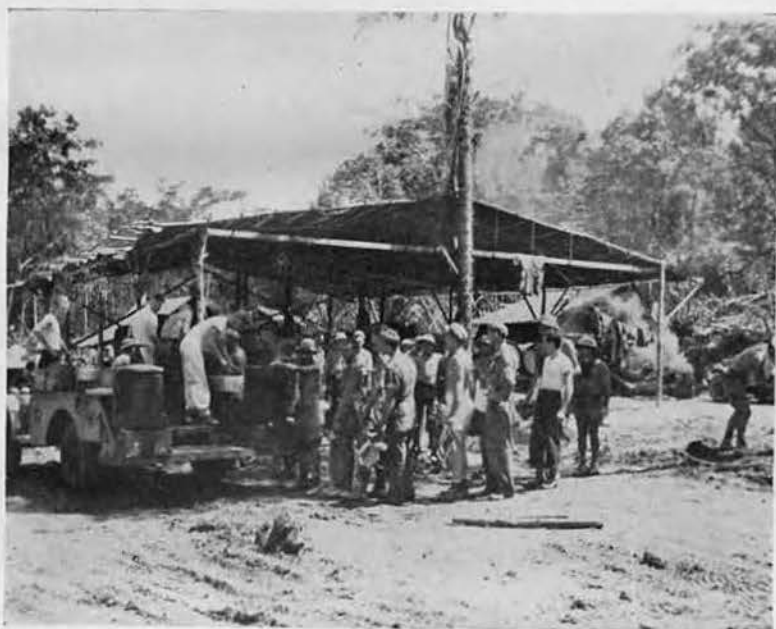
CHOW WAGON visited strip and adjacent shop areas on rigidly fixed schedule until Stirling Field was completed. Working eight-hour shifts—three shifts spanning 24 hours—the men had just enough time off to eat on job.
