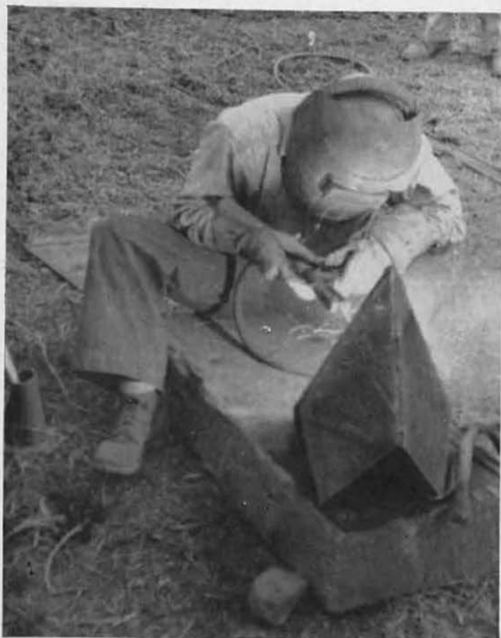
SHOEMAKER. Frequent solid-rock ledges in river beds presented formidable obstacles to pile-driver. Only after pointed shoes of steel plates were fashioned together and attached to the leading end could piles be driven home. Tom Clements is welding.
