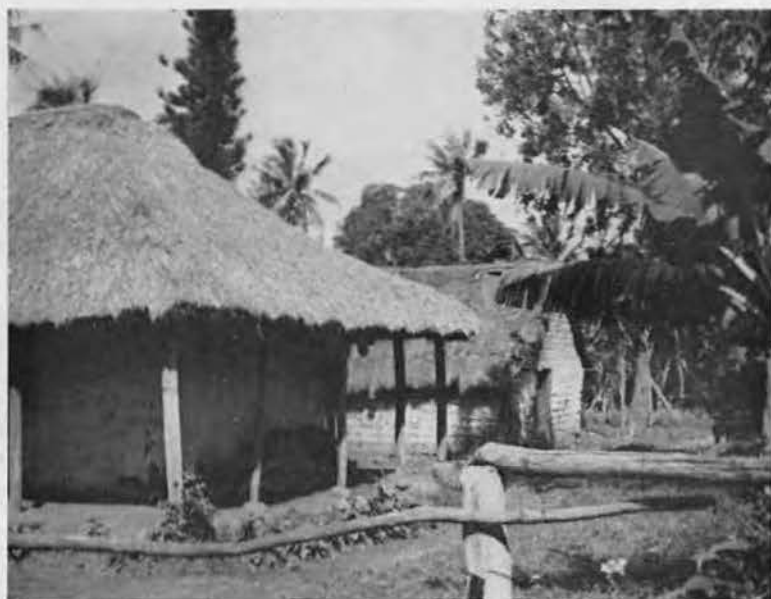
HOME, SWEET HOME. Besides providing an adequate shelter against the rain, straw-thatched roofs of native huts were a haven for rats, snakes and insects. Walls were mixture of clay and earth, but kept the temperature inside quite comfortable.
