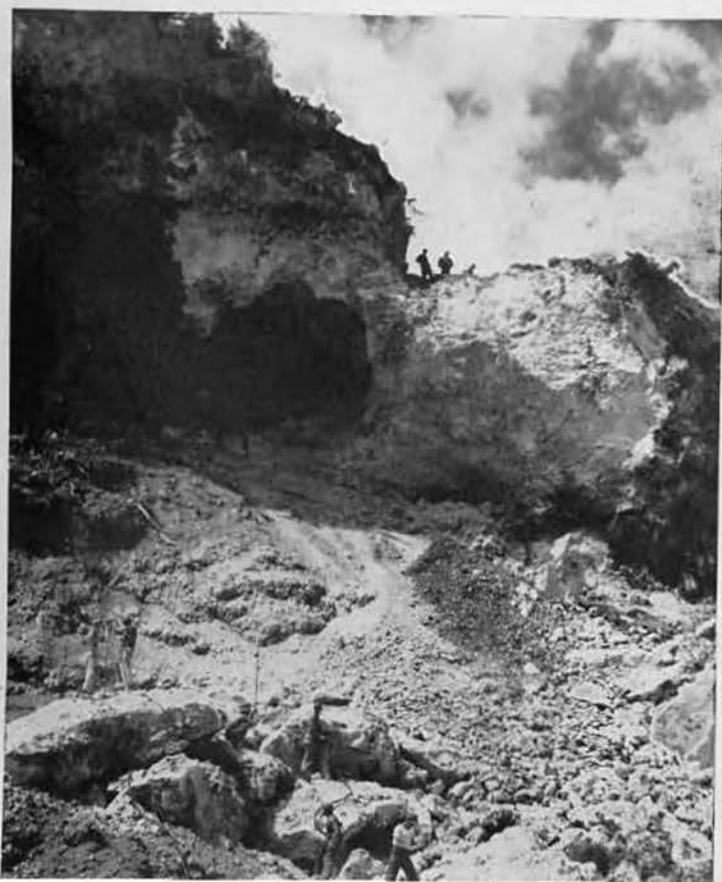
DEATH SCENE. Demolition gang is drilling holes for charges to reduce size of boulders. At this spot, Dale Anderson was accidentally killed and Dick Henry seriously injured on 24 August. Neither are in this group as they worked opposite shift.
