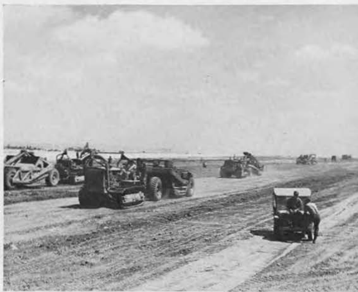
HUDDLE. Lieut. Ben Markette (seated on jeep), battalion transportation officer, discusses the general state of affairs at Yontan with Lieut. Louis Spaw, who is overseeing engineering aspects of rush project. Already 4,500 feet of sub-grade are finished.
