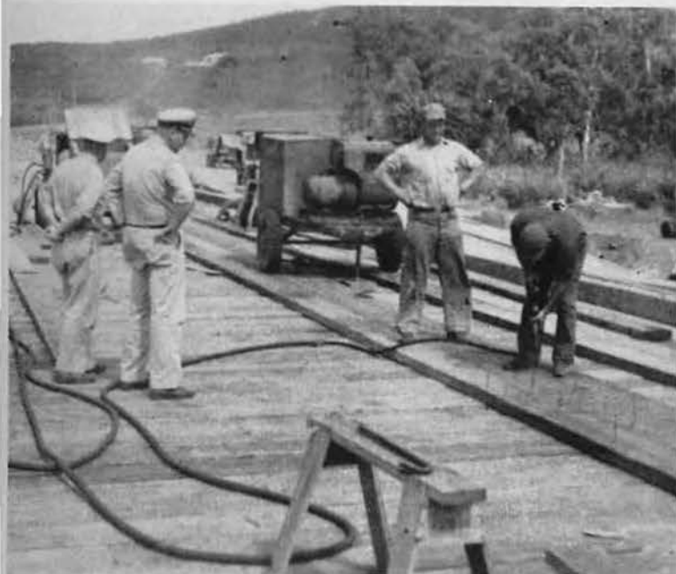
GOLDEN SPIKE? Four lanes of heavy top tread were eventually added to save wear and tear on the main decking of bridge. Chief Bill Inness, Lieut. Ray Pape and F. K. Jones observe as J. C. Jones drives a final row of spikes.
