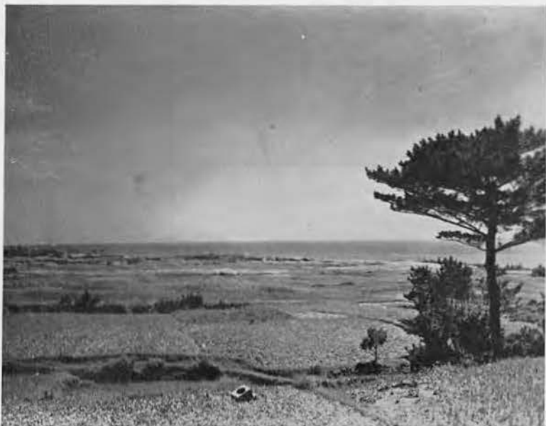
BEFORE CONSTRUCTION commenced, the general site for the new airfield looked like this. This view was taken looking southwest toward the East China Sea and famed Green Beach where Americans made initial Easter Morning landings.
