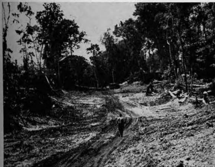
WIDE CLEARING, made for a main highway on Stirling Island, has been brushed out below airfield. Odd-shaped New Zealand truck was used by a Kiwi field bakery in delivering bread to various outlying units. Early roads weren't too good.
