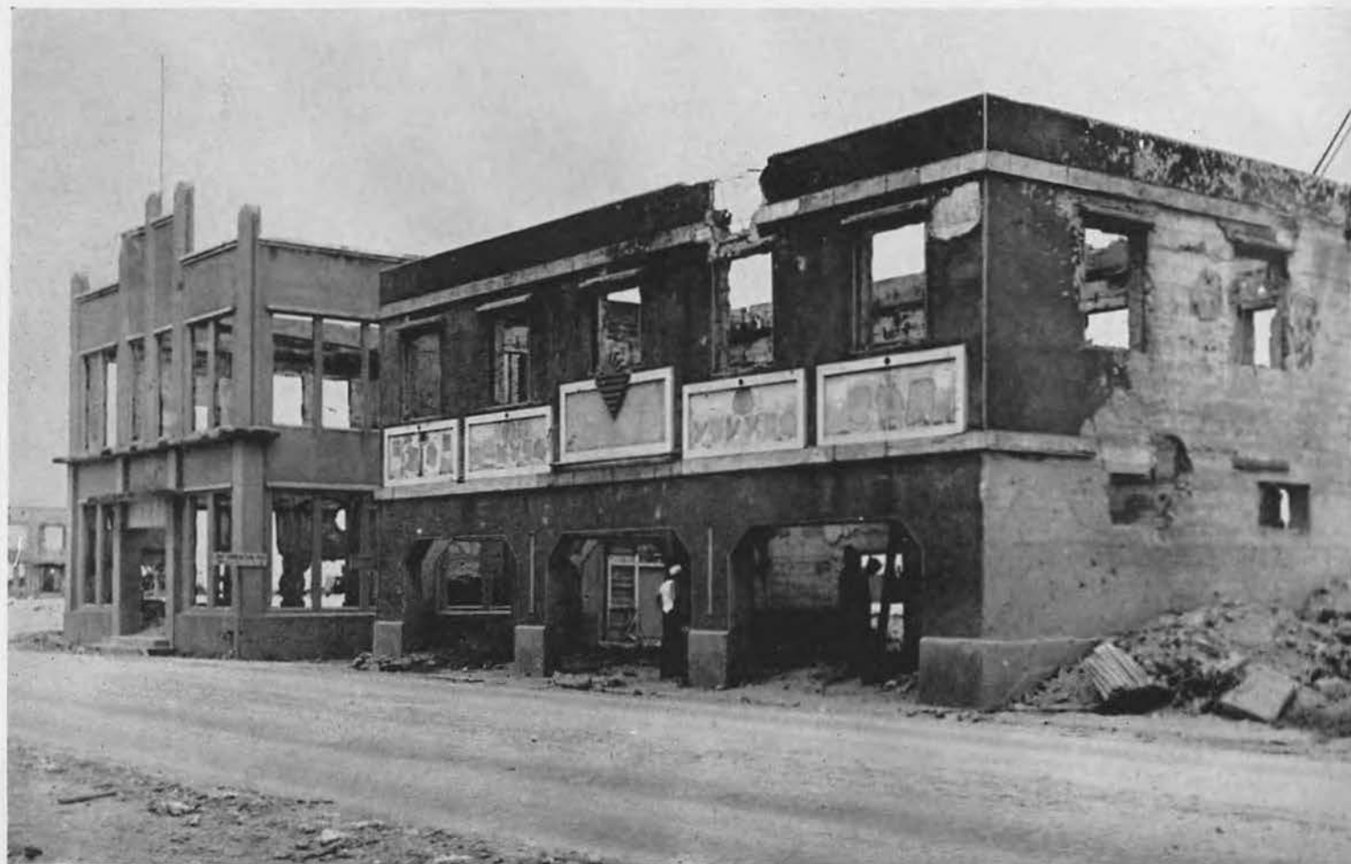
BUSTED BANK. With windows, including frames, completely blasted, roof gone and walls peeling, all that's left of the once proud Bank of Garapan stands as grim reminder to Jap survivors of U. S. might. Yawning hole at top-front of building and those in right end indicate direct hits by giant
