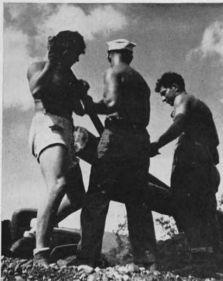
BULLGANG. Roughest and toughest crew on Bourail job was Chief Frank Rychlak's "devil-may-care" bullgang. These huskies threw trailer-loads of heavy timbers around with ease of lumberjacks. Above: Eddie Breitenbach, Leo LeBlanc and Phil Mungiole.
