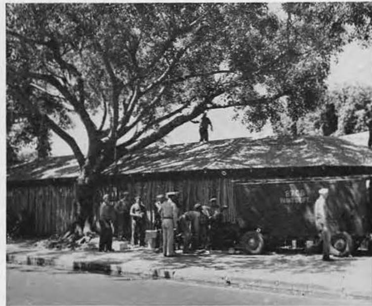
SPRAYING, INC. The 87th paint crew eventually became a rather familiar sight along Noumea's busy streets. Chief Cedarstaff's crew of experts mixed and prepared color mixtures on the spot with this mobile unit. All paint was applied with spray guns.
