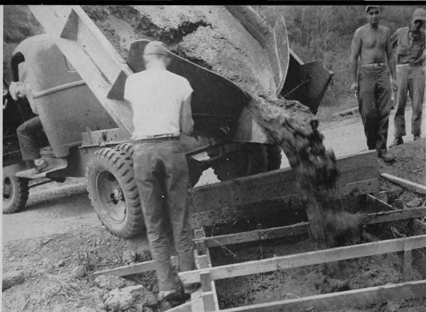
POURING THE MUD. Once the oil-drums were fashioned together and the supporting forms built, mixed concrete was driven up in trucks whose beds had been somewhat redesigned and poured through a rear chute. Mike Kocian and Raymond LaRue (right) stand back from wildly splashing
