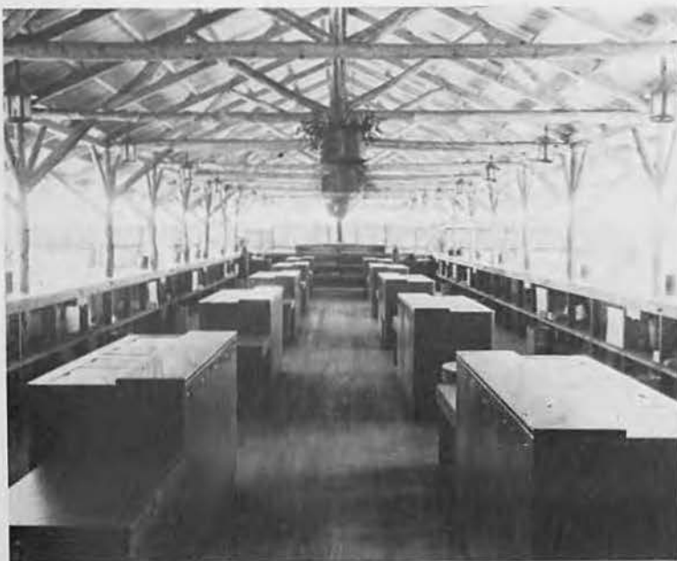
WELL DONE. Ten sizeable coolers in interior of completed fountain assured thirsty GIs of iced beer and coke. More large reefers in surrounding buildings kept reserve supply of beverages at constant temperature.
