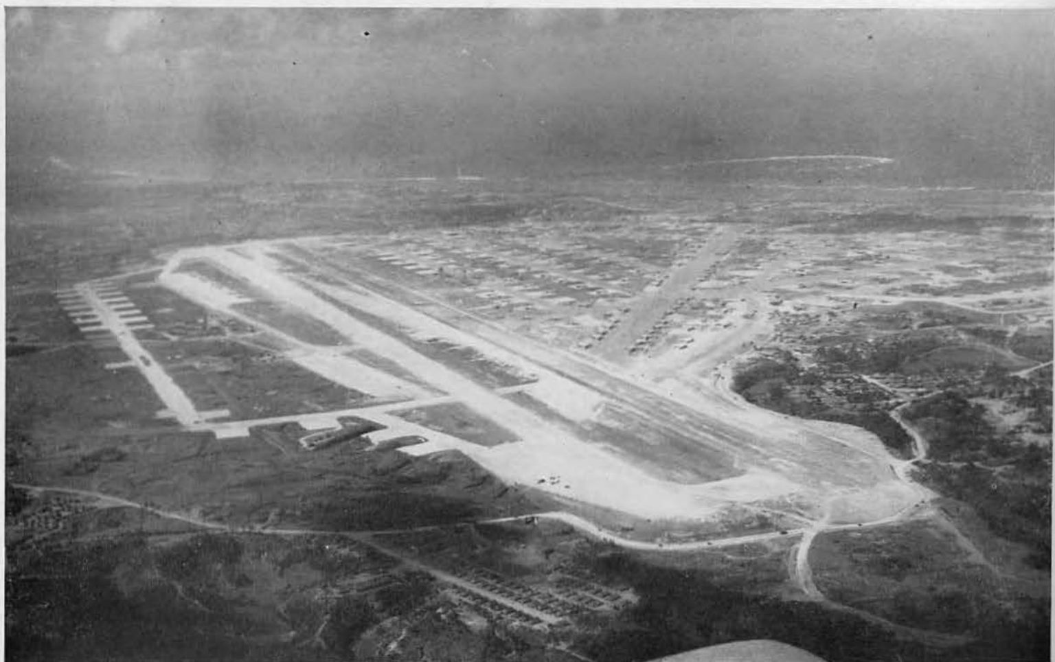
YONTAN COMPLETE. This aerial view, taken several weeks after the battalion finished its work, reveals the immensity and completeness of the overall Yontan installation. The 87th-built strip is the dark runway extending from right foreground to left center. Black-topped with asphalt,
