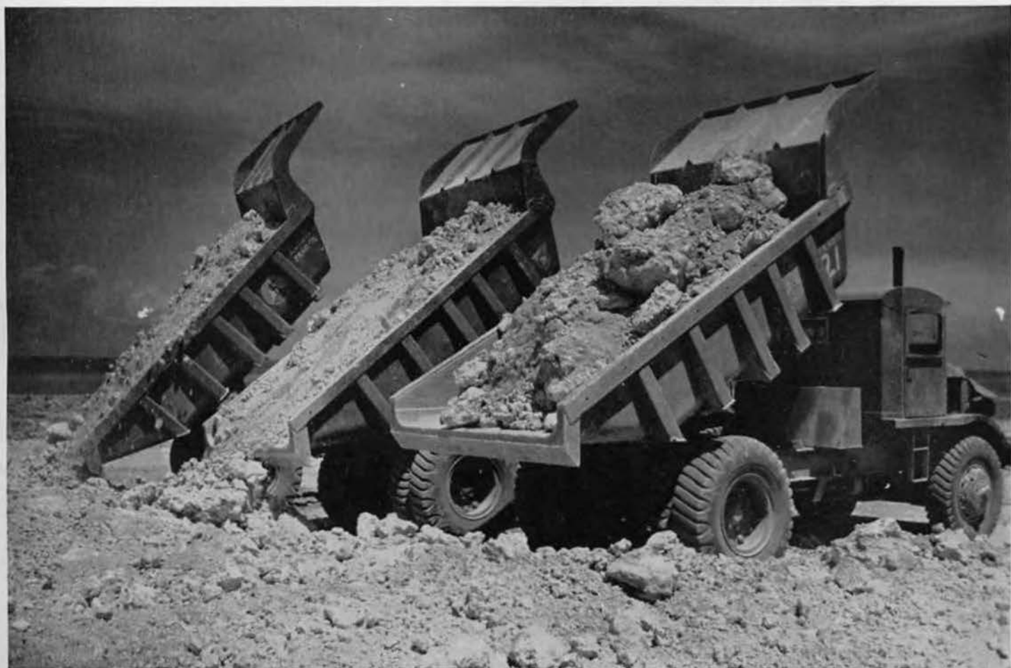
IN FORMATION. Three monstrous Euclids simultaneously dump 30 yards of paving coral onto strip at a single clip. This would be enough material to pave an area of runway three feet long and 200 feet wide. These three "Ukes" were piloted by Lyman Dailey, John Radel and John
