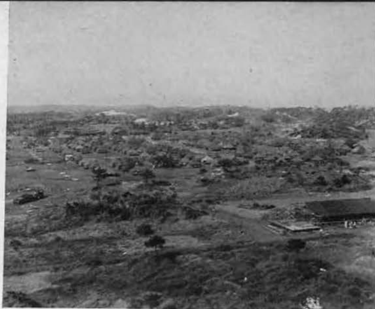
BATEN-KO Camp. In September, the Army finished taking over Bolo Point and the 87th was forced to move to Baten-Ko, near Buckner Bay, where they moved into the partially completed camp recently vacated by the 66th Seabees.
