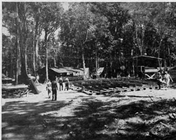
HIGH COMMAND. Beyond movie area is an overall view of battalion administration offices. First long structure housed Post Office, Personnel and Disbursing. Tents further along accommodated: Labor Pool and MAA Offices; OinC and Exec headquarters; and the Supply Office.
