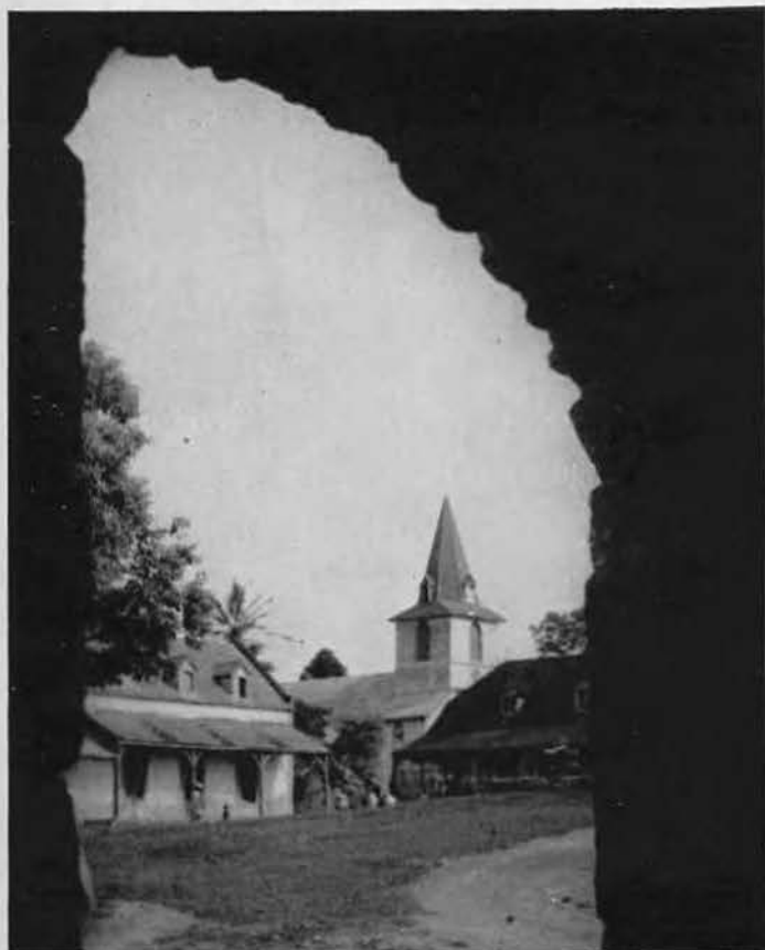
ST LOUIS MISSION, with its rich mixture of the medieval and the primitive, drew hundreds of incredulous Seabee visitors. The mission church, seen here through a massive archway, was built by native Kanakas under guidance of missionaries, who also helped.
