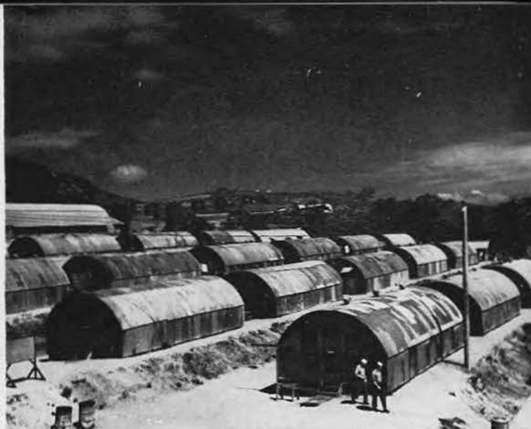
SEABEE HIVES. It was only a matter of days until almost everyone was comfortably settled under metal roofs. Located on a sharp slope, the rows were first terraced to keep the huts on an even keel. Officers Country is in background.
