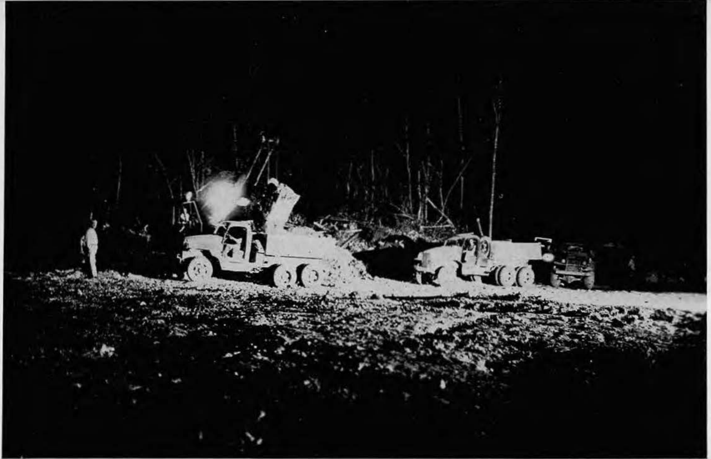
DAY AND NIGHT. The equipment didn't shut down until it broke down unless Jap bombers came over. This was a quiet night with everything running smoothly as the stripping operation progressed. There were four spreads like this clearing at the edge of the
