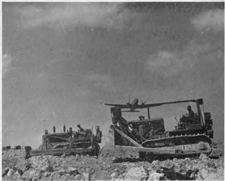
TOKYO TROLLEY. A Curtiss Commando of the Air Transport Command (ATC) takes off on a run to a rear base in the Marianas. Max Mathas on TD-18 (left) and Gene Ross on D-8 trim off edge of the pavement as the work progresses.
