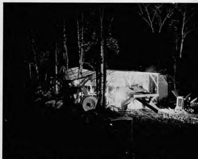
CASUALTIES. The welding shop was part of the equipment "sick bay." The going was tough and it wasn't always the coral that moved. A pan pulled out of shape and a rooter hitch pulled apart are being "treated" by welders.
