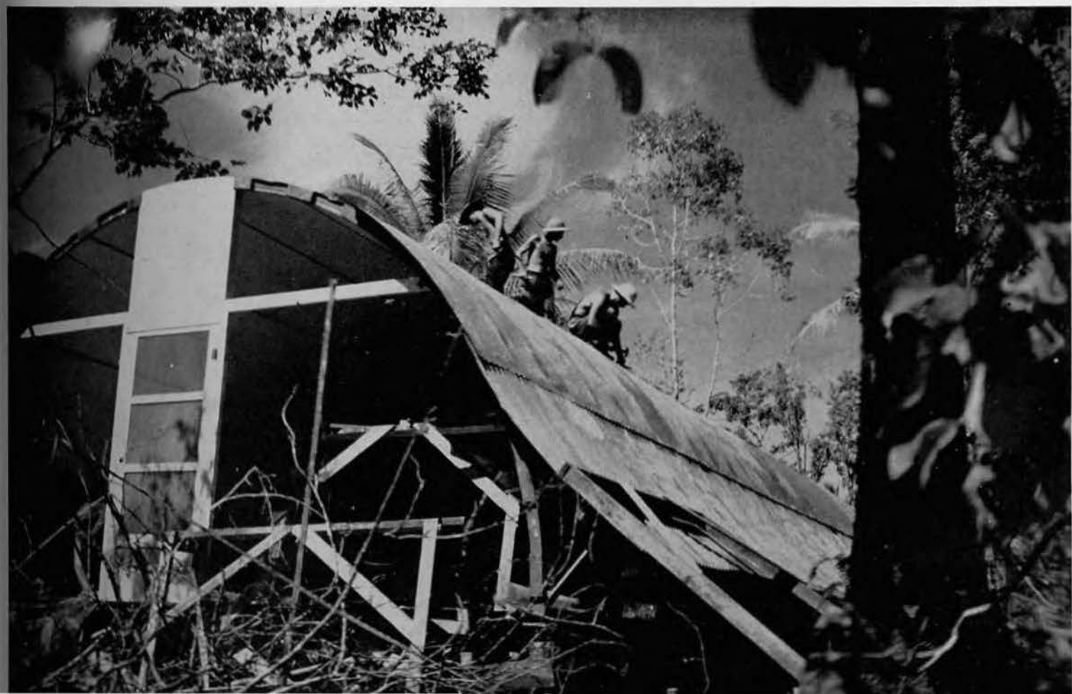
JUNGLE HOSPITAL. The first quonset hut erected on GOODTIME nears completion as a few carpenters work aloft while others finish inside trim. A group of these huts—eventually manned by medical officers and corpsmen—served as an emergency hospital for all air strip personnel. Airfield
