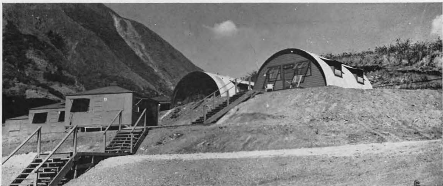
TOP OF THE HEAP. Comdr. Easterly and Lt. Comdr. Flynn occupied the three-room quonsets shown on upper terrace. The breath-taking view from this highest level surpassed all others in the area. Equipped with run-
