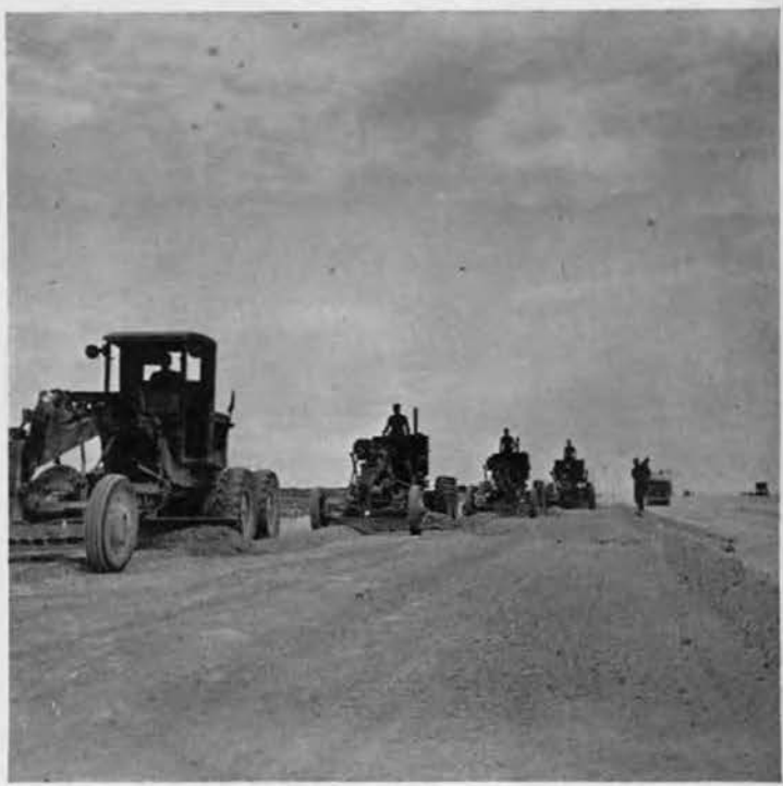
DOWN THE LINE. Four of battalion's five motor graders are snapped in echelon as they carry a nice windrow of good looking coral. At the controls (left to right): C. J. Rominger, Chester Watkins, Chester Pope and Sam Newman.
