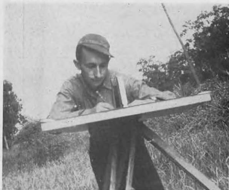
TOPOGRAPHER. Jean Worley of Lincoln, Nebraska, pores over his plane table to plot the topography of one of the multiple bridge sites and culverts, which were built along 13-mile stretch. Worley sports typical cap worn by most Seabees overseas.
