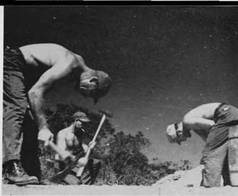
SMOOTHIES. Final touch to the bridge was smoothing off rough, uneven planking and rounding off end approaches. Here, men revert to use of time-honored adze, which in hands of such men as Gordon, Lingle and others, gets results.
