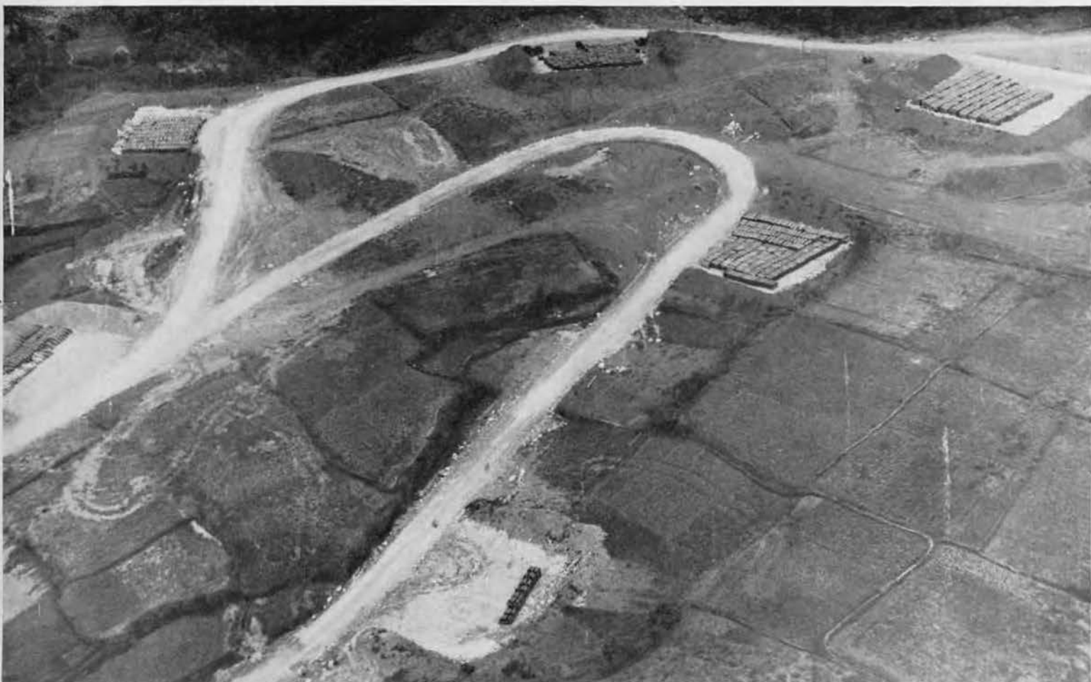
FROM ABOVE, a comparatively small portion of Yontan bomb dump is seen in this aerial view taken in May from a Piper Cub. Actual sections are quite well dispersed and reveted to prevent spread of fire in case of direct bomb hits. This shot reveals fairly good detail of how native
