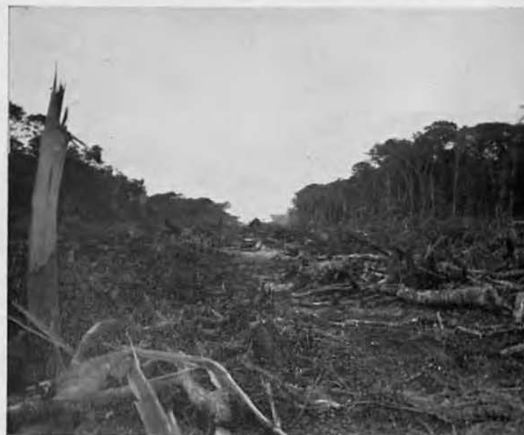
AFTER THE STORM. 'Dozers, timber-cutters and blasting crews create a real tangle. Chief Bos'n's Mate Frank Rychlak and gang are busy loading logs, using cant-hooks and a stirrup puller. 'Dozers then pushed remaining branches, stumps and foliage to sidelines.
