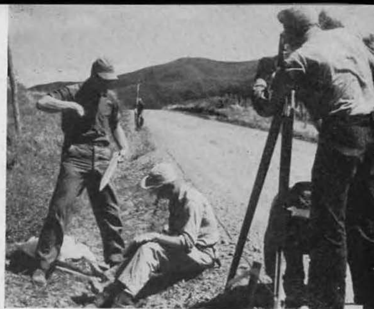
ON LOCATION. With eight projects in progress simultaneously, the battalion's two survey crews had more than their hands full in keeping a jump ahead of the hustling construction gangs. M. O. Brenn reads transit data off to Chief Paul Sowers (seated).
