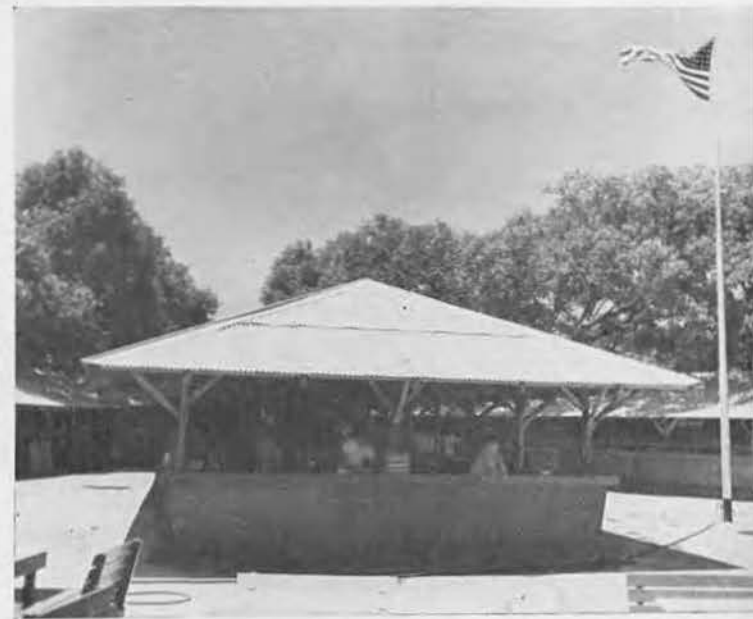
ALL SET to open next day (Thanksgiving), exterior of TRADE WINDS fountain was finished with stained plywood and a fireproof asbestos roof. Once opened, its 175-foot bar was never without several hundred parched servicemen.
