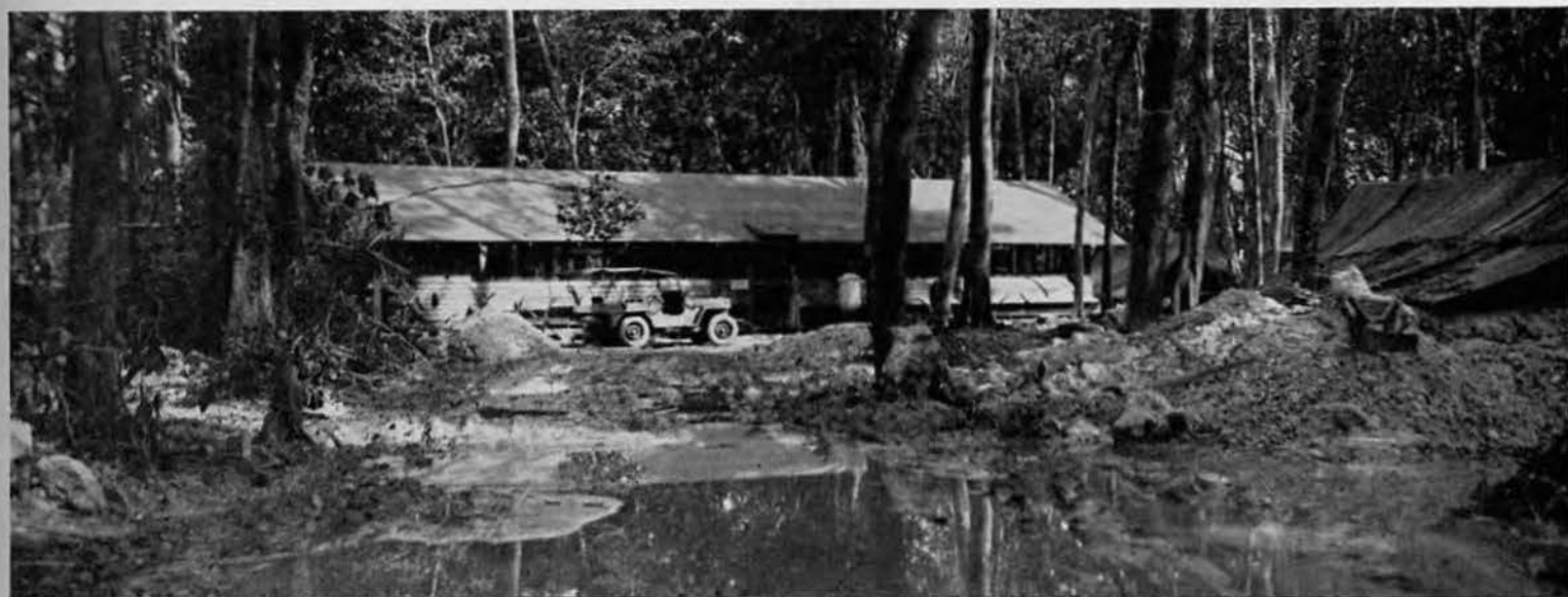
TROPICAL HOSPITAL. In this rain-drenched jungle rendezvous, safe from the probing eyes of enemy bombers, the Sick Bay was constructed none too soon. Here, near a high cliff overlooking the gleaming Coral Sea, top-
