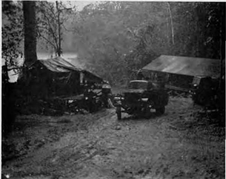
WATER POINT. In the midst of this God-made jungle, a Seabee-built (87th) water plant is operating. Trucks haul the precious fluid continuously so sweat-soaked men—to whom a bath was only a memory—may again feel human. Water rated a top priority.
