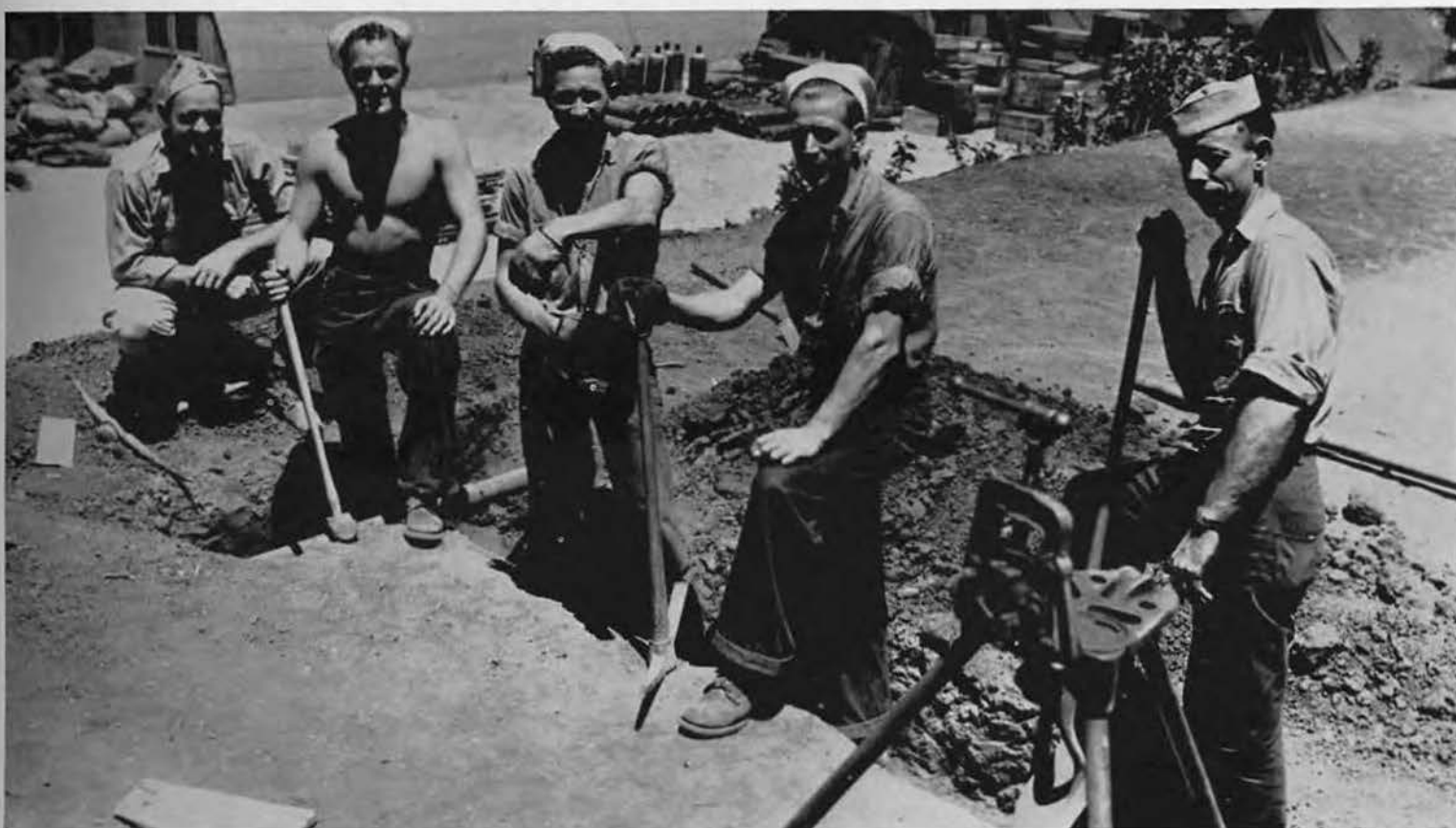
NOT IN THE CONTRACT. Battalion plumbers were truly "jacks-of-all-trades." Besides piping the entire camp for showers and plumbing Sick Bay, mess hall, laundry, etc., they frequently had to dig their own ditches
