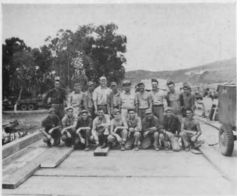
BRIDGE BUILDERS. Most of the credit for construction of seven fine bridges on tough Bourail job must go to Chief Inness and the 18 stalwarts of his hustling carpenter crew. Here, the entire gang knocks off for a group portrait.
