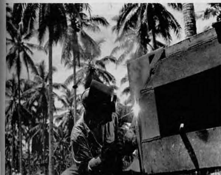
ON TARGET. Vernon Jacobson welds on a section of pontoon. Seabees had put pontoons to many ingenious uses, but none more unusual than this unit. Upon completion, this one will serve as an oven for the bakers.
