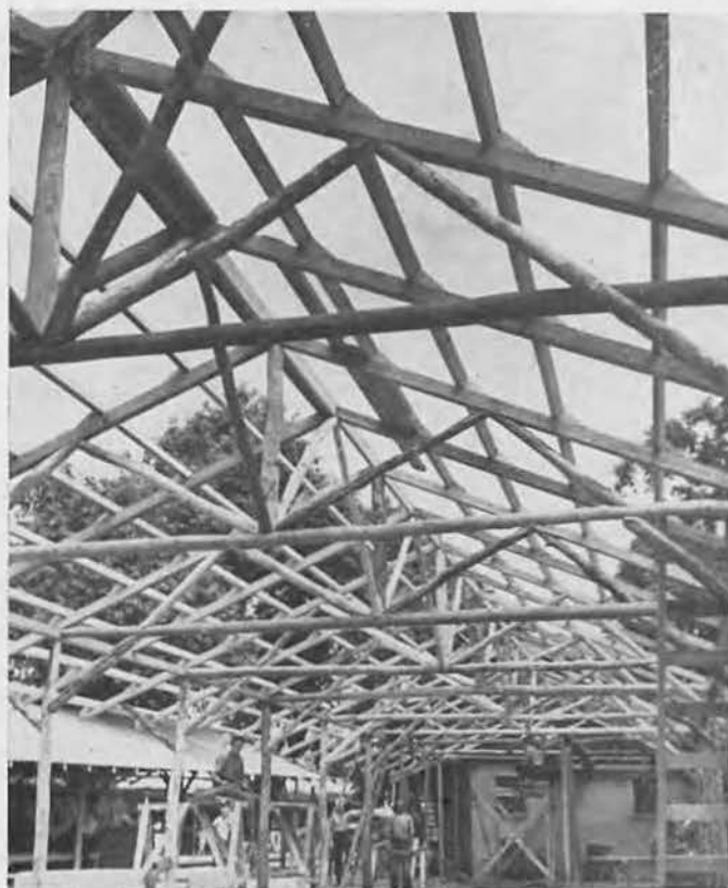
RUSTIC UPHOLSTERY. Framework for all structural work in compound was of native rough timber and a minimum of finished lumber. Project was stymied time and again for lack of sufficient building materials. Here, construction was still in progress.
