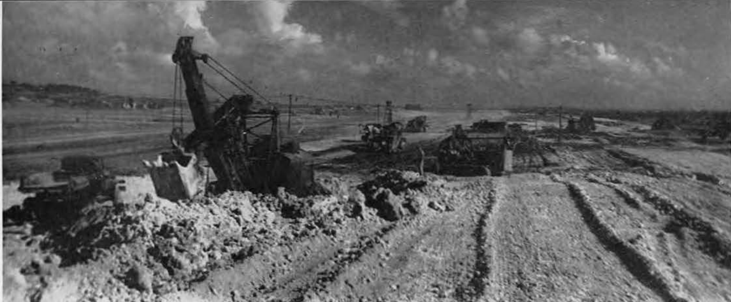
DOWN THE MIDDLE. A 2½-yard shovel digs handy paving coral right out of the middle of what will soon be a B-29 runway. This particular hill furnished enough coral to completely pave the first 3,000 feet. When this spot was leveled to grade, a new coral pit was opened nearby,
