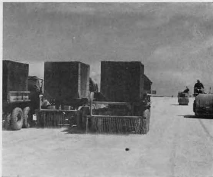
GETTING SALTY. Sprinkling and rolling of the glazed runway continued day and night as the completion of the project neared a record breaking end. Three of the battalion's four water sprinklers wet down surface with salt water.
