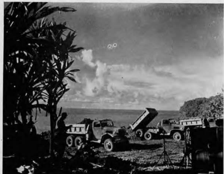
GETTING RID OF IT FOR KEEPS. Gushion E. Bolt supervises from the shade of a convenient tree as trucks dump loads of strippings into the sea some 80 feet below. Most stumps and roots were disposed of in this manner—once and forever.
