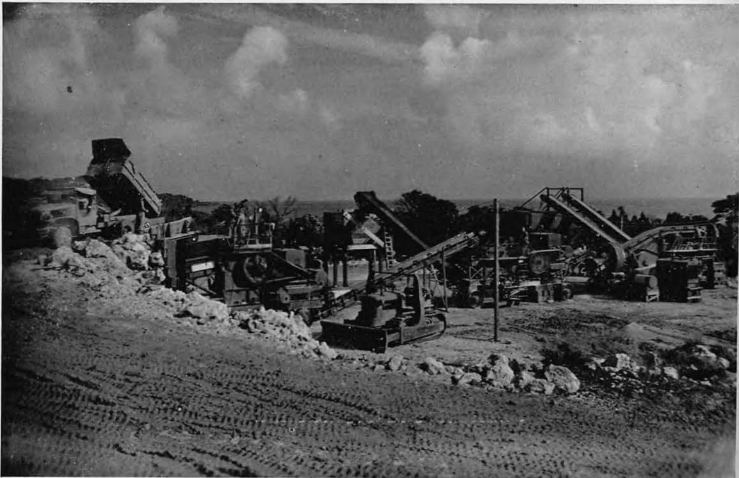
ACCENTUATING THE MAXIMUM, the fully completed Nagahama crusher grinds away without a hitch as the enormous jaw crushers chew up boulders of all sizes from the nearby quarry. Twenty-seven tons of dynamite were
