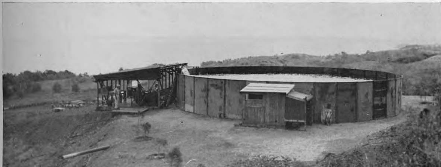
SOME CONTAINER! One section of a 10,000-barrel, bolted steel tank used as the water storage point for entire camp. Planned by Carpenter
