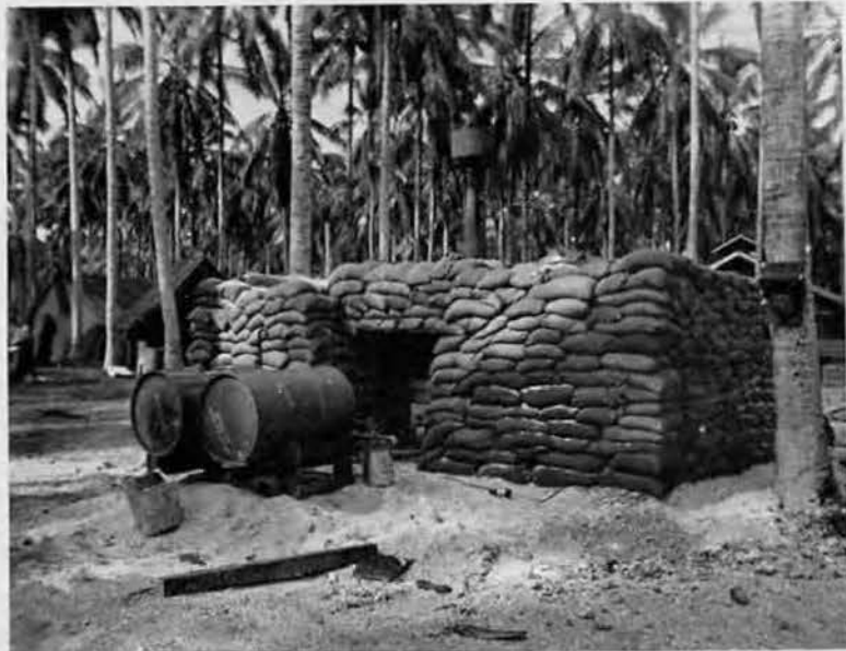
OUTDOOR OVEN. The finished oven is well insulated with sandbags to maintain the high temperature necessary in good baking. Despite its unusual appearance, the oven successfully provided the always hungry 87th with all-essential bread and cake.
