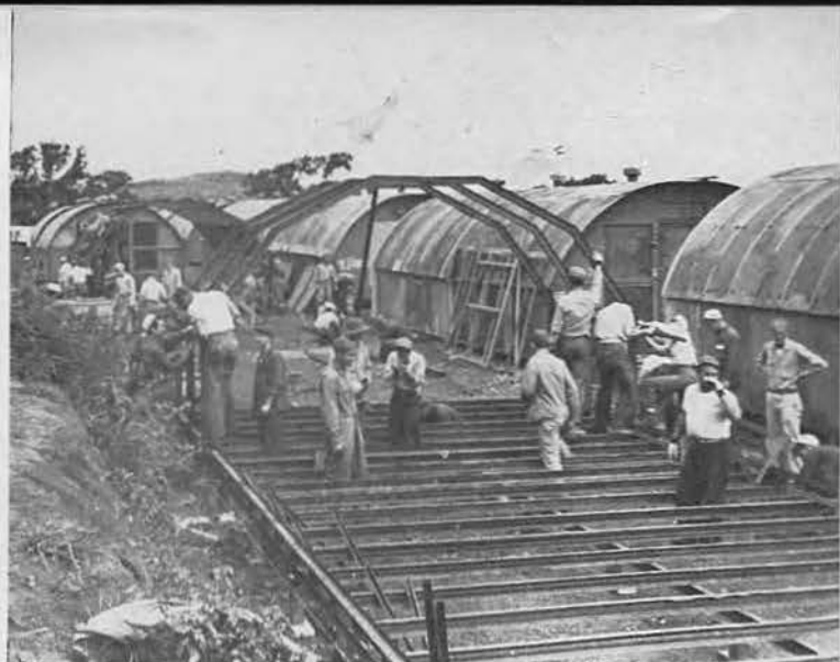
ASSEMBLY LINE. Four quonsets every eight hours was the record set by the four carpenter crews of 10 men each. Here, Chief Sam Beacom stands by as the arches are being hoisted into place on the steel-ribbed foundation.
