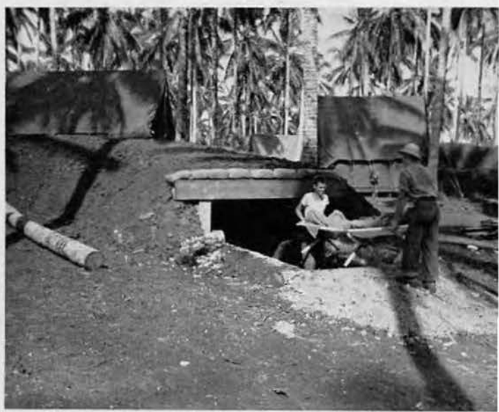
ALL CLEAR. Pharmacist Mates Fred Colby and Gaylord Hold remove a "patient," Archie ("Red") Reynolds, from roomy Sick Bay dugout after a simulated air alert. This sturdy shelter, built to accommodate 16 beds, was reinforced by heavy timbers and sandbags.
