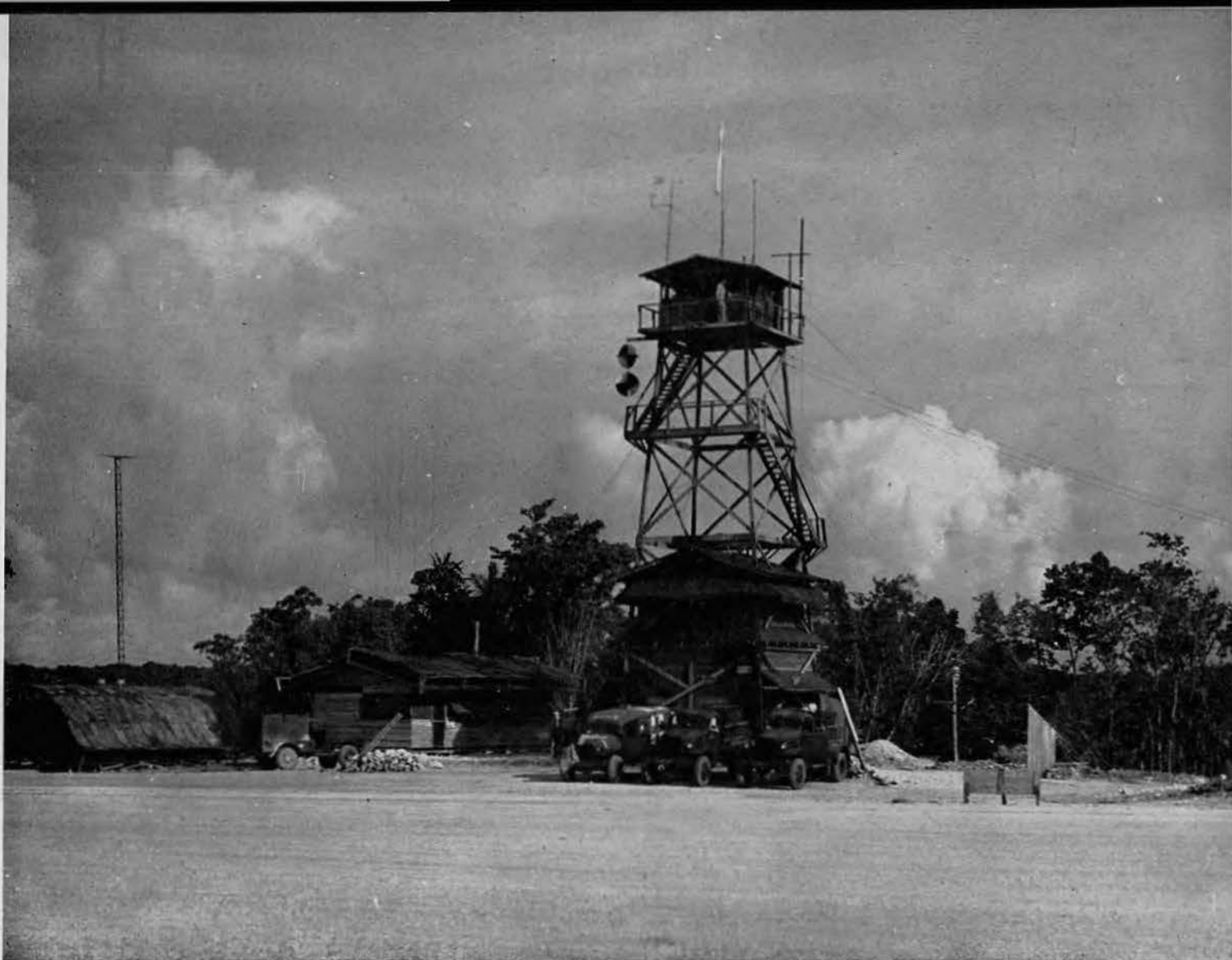
CENTER OF OPERATIONS. Not only did the Earthmovers build a strip on Stirling, but they constructed aviation facilities to go with it like this 60-foot control tower and the communications and weather huts shown here. Equipped with sizeable bolts and timbers,
