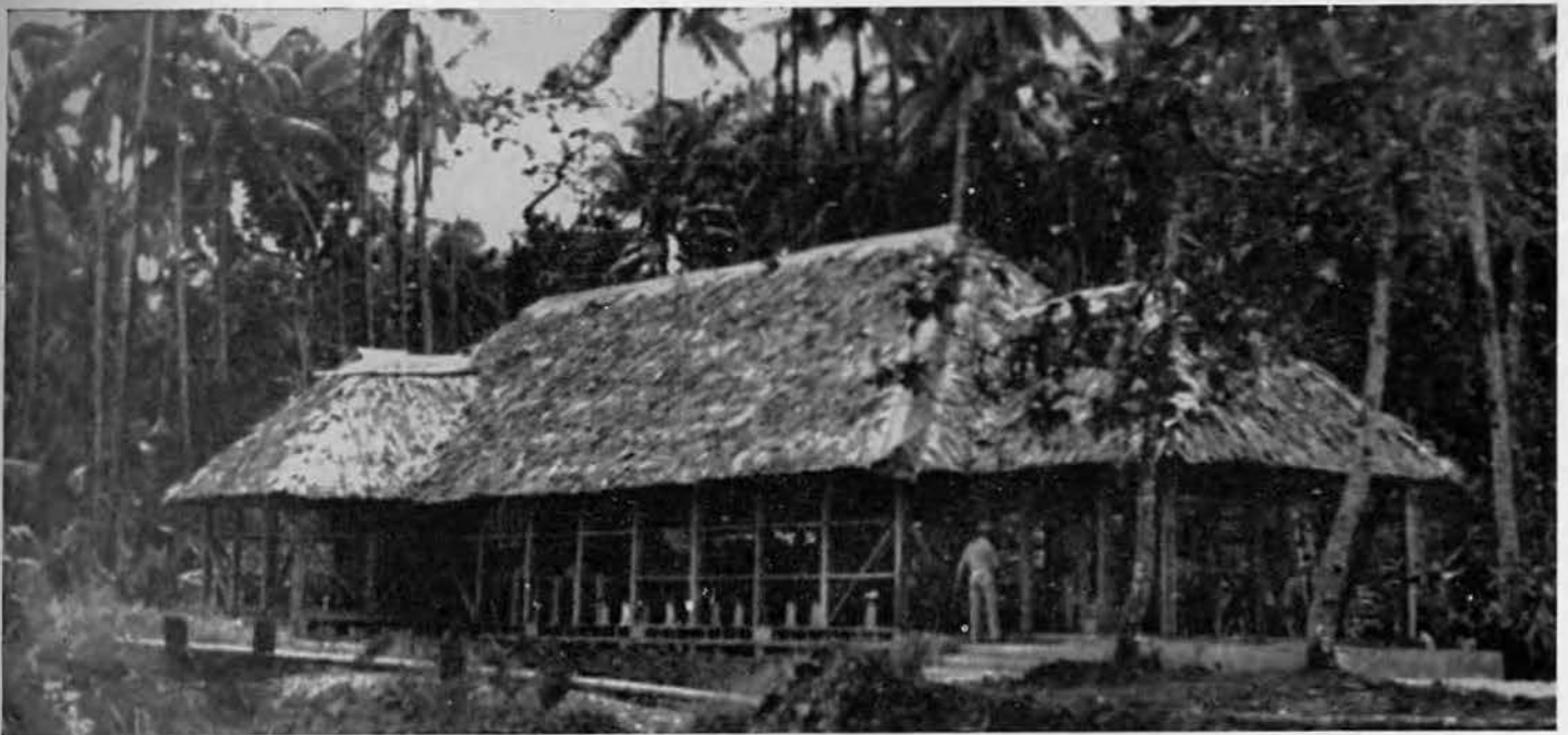
REPARATION. With peace eventually restored in the Treasuries, New Zealanders and Americans—as reparation for destroying the native church in exterminating the enemy—began building another church for their island friends. New edifice was erected on a beach in vicinity of former church site. Structure featured ornate windows
