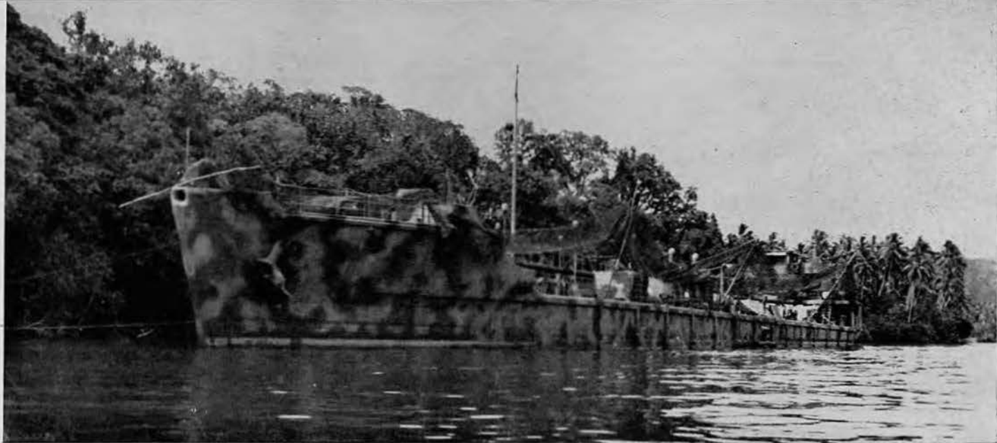
YOGL gets camouflage job from Chief Vic Cedarstaff's paint crew and riggers. Two of these huge aviation gasoline storage barges were stationed in Blanche Channel and they needed to be disguised. Chicken-wire netting with strips of green fabric interwoven was suspended over vessels in uneven
