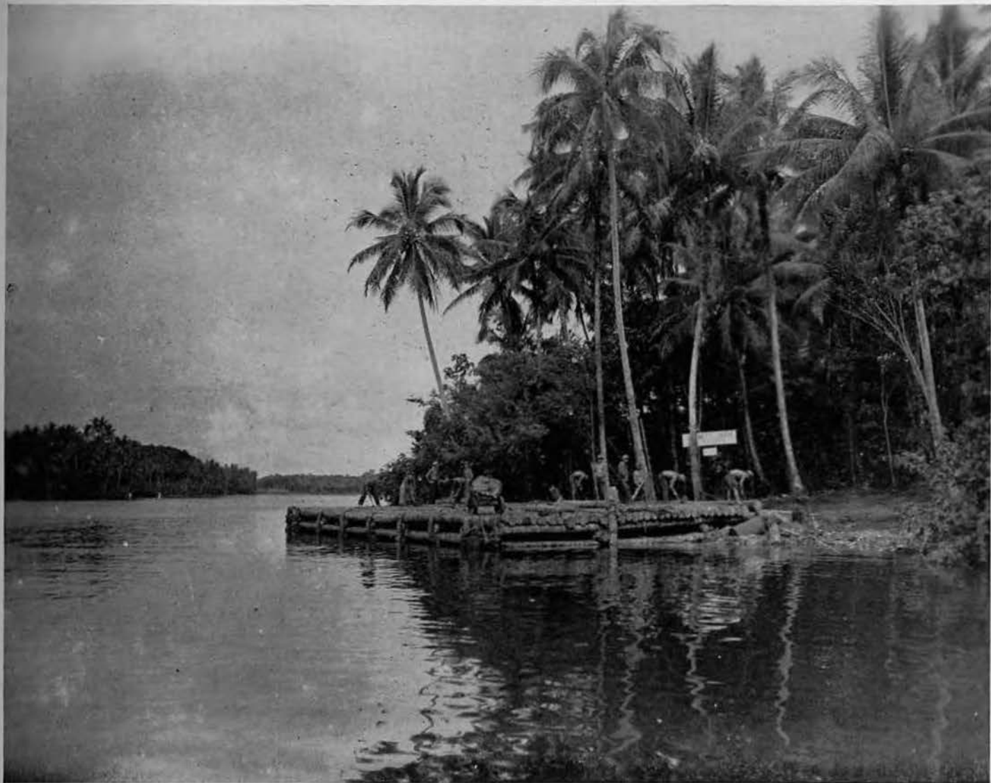
PT BASE. Torpedo dock for the cocky little night raiders was built by Chief Bill Inness and his Company A carpenter crew. Working long days with only hand-axes, this group completed the first Stirling project assigned the 87th in jig-time. Made of lashed coconut logs, the above crude struc-
