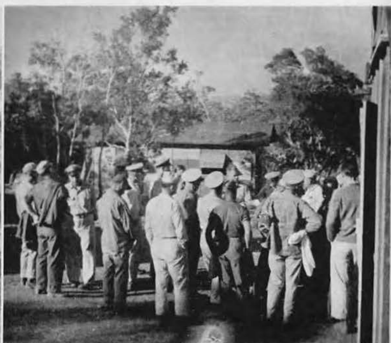
HUDDLE. An important part of the daily work routine was the morning pep talk to crew chiefs by Lieut. Pape. Here, the past day's work was reviewed and orders given for the new day's construction program. Attendance was mandatory—and without fail!
