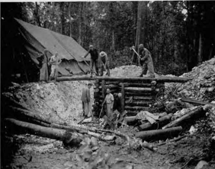
NERVE CENTER. It was first things first in constructing the new camp. Here, axe-swinging carpenters build bomb-resisting underground communications dugout, using watersoaked mahogany and teakwood logs from surrounding forest. Structure was eventually sandbagged.
