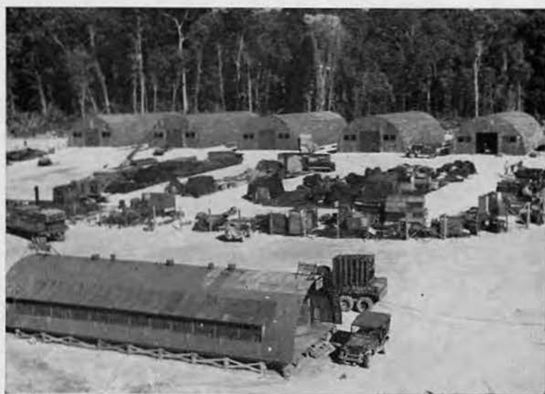
SUPPLY DEPOT , built in dock area, consisted of five 40x100 quonset warehouses and a compound surrounded by a barbed-wire fence. Office of Port Director was the 20x48 quonset (foreground). Area was once a Seabee baseball diamond
