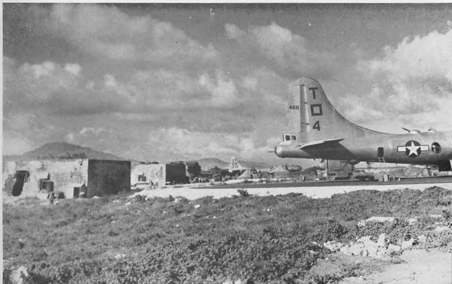
CRAFTSMANSHIP. Mute tribute to the uncanny Jap craftsmanship was found in these concrete pillboxes lining the southern ridges of Isley Field. Walls, three-foot thick, remain intact despite terrific Naval bombardment and aerial bombing during the invasion. When the air corps took over
