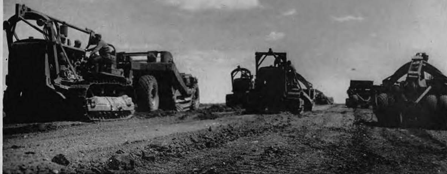
MASS PRODUCTION. A typical heavy yardage spread, pans in this shot often moved 900 yards of Jap earth per hour. With the work carried out in above grand manner, it is easily understood how Yontan was completed in such gratifying time. Using only the
