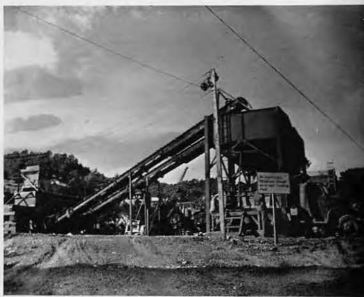
STORAGE BINS for crushed stone (right) feed materials into trucks that haul it to various projects. These bins are filled by means of conveyor belts (left), which are driven by crusher motors. No unauthorized personnel were allowed.
