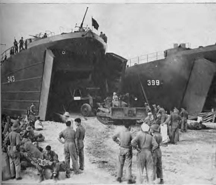
CATSKINNER. J. B. McLelland backs his loaded carryall through the yawning doors of LST 343. Heavy equipment went on the well deck, while trucks and jeeps were parked topside. Frank Keker (left foreground) calmly reads "Superman."
