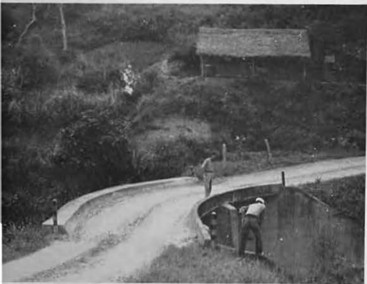
INSIDE CURVE. In sharp contrast to modern road and bridge construction methods of Seabees were the primitive, hand-made efforts of the native Franch. Lack of equipment and proper materials, coupled with different ideas, resulted in this curved curiosity.
