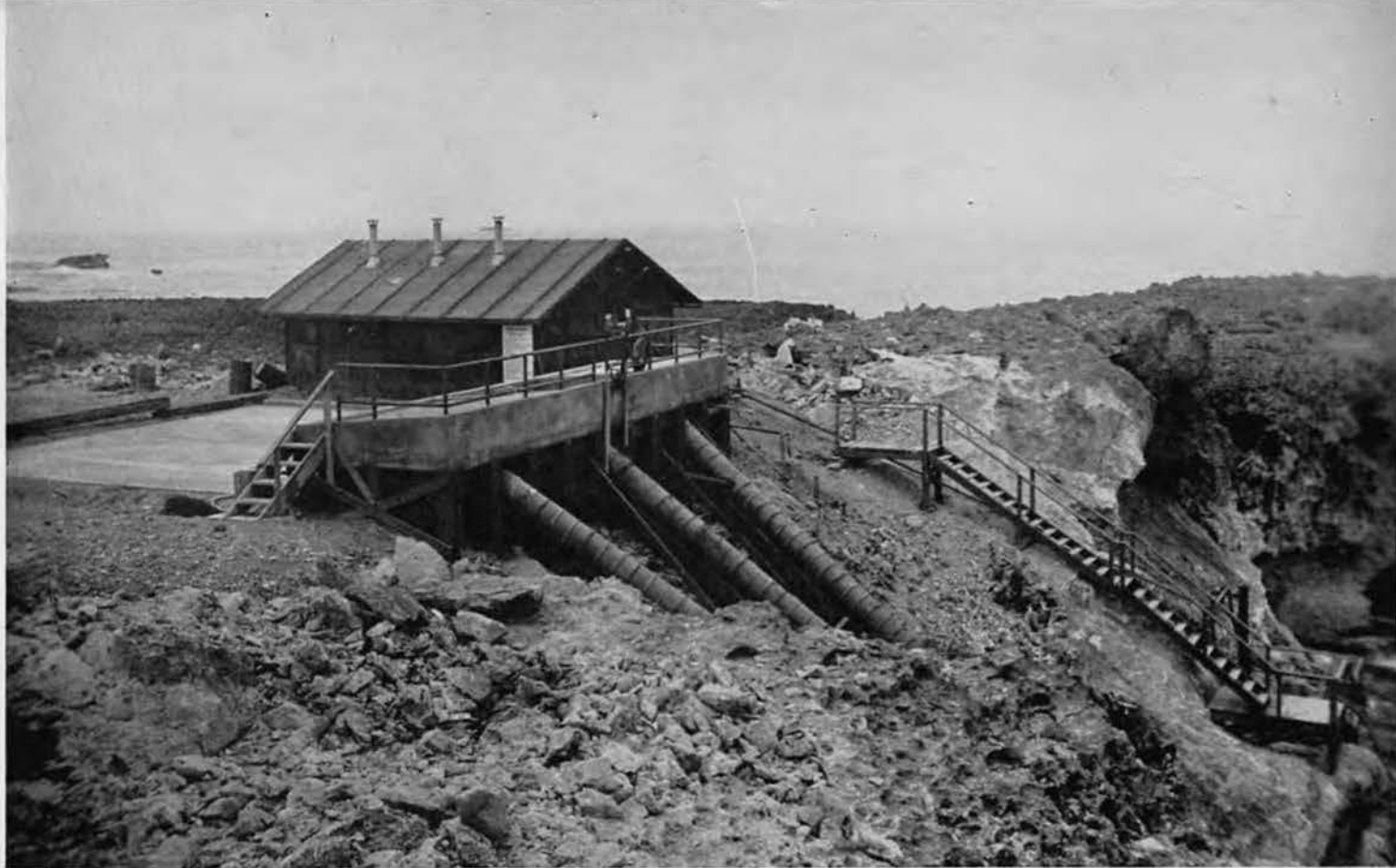
SEABEE WAY. Construction of Bolo Point garbage disposal plant required the collective skill of nearly every 87th division before completion. After a 'dozer clearing by Transportation, R and S demolition crews blasted proper slope angle along cliff. Carpenters then erected boiler house
