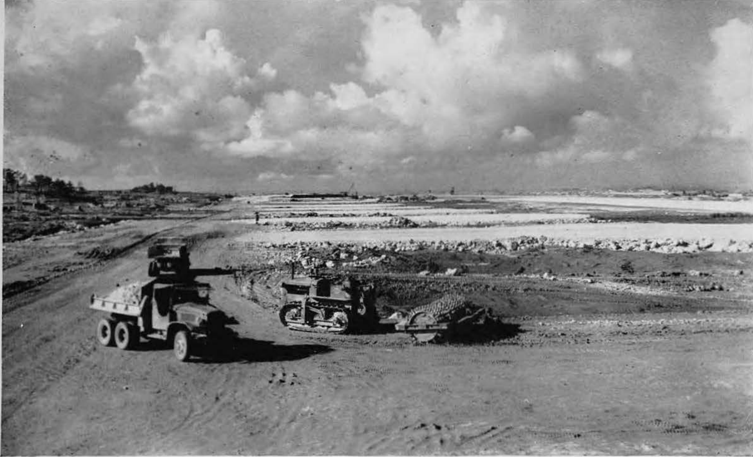
COMING AND GOING. An empty truck heads back to the pit for another load of coral as a full vehicle turns into a hardstand to dump its burden. This is a general view of unpaved taxiways and paved hardstands looking south. Bolo Field proper is at right. Sheepsfoot roller (foreground)
