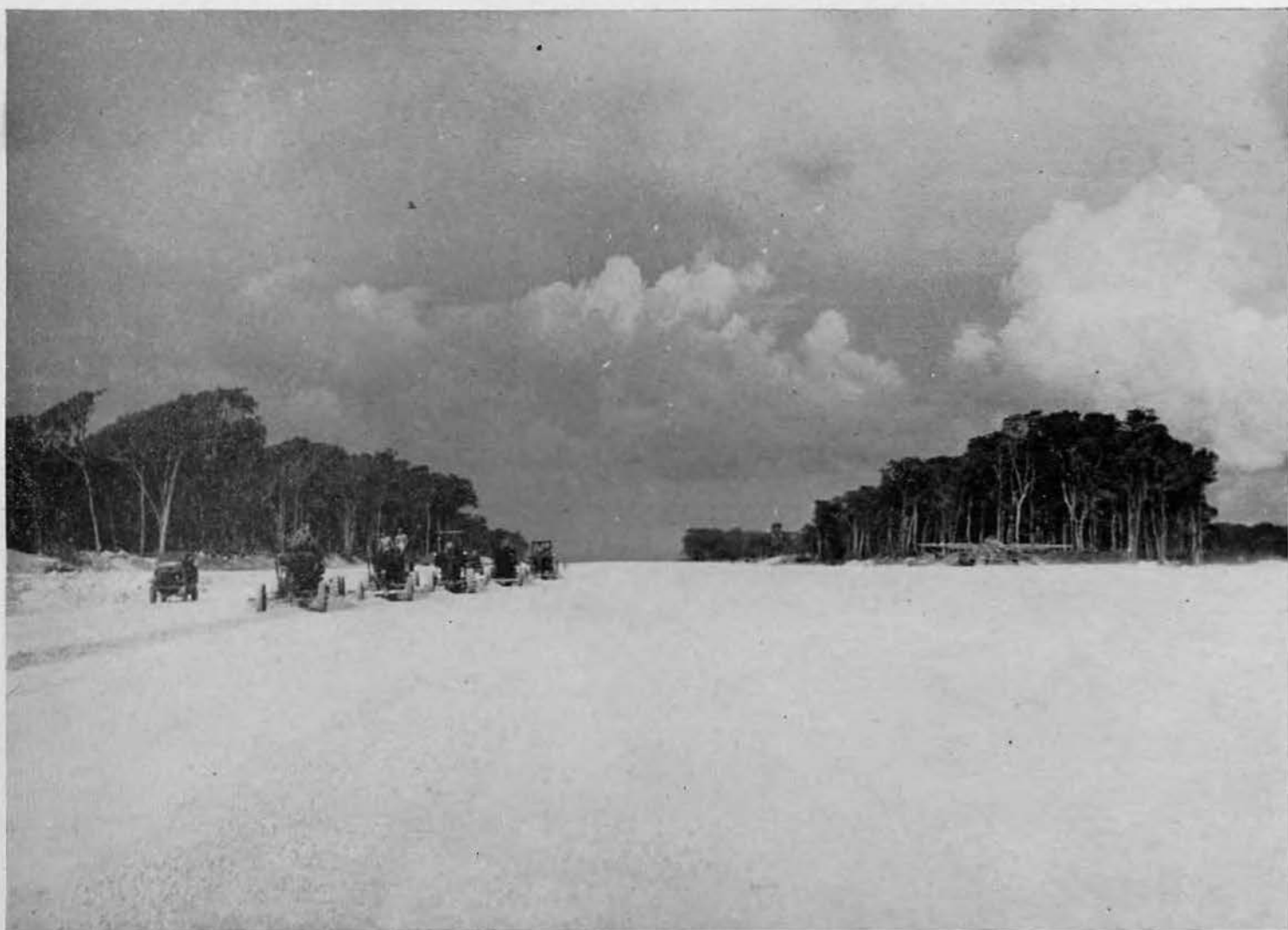
CUTTING A WIDE SWATH. The Earthmovers always tried to observe a basic rule: "Never spread yourselves thin." The attempt was made to tackle every phase of the job with sufficient men and equipment, well grouped for close supervision and balanced operation. Here, the finishing spread illustrates the 87th's favorite method of concentrated attack. Not plainly visible are the salt-water spray trucks and rollers following the graders. The
