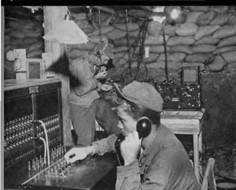
NUMBER, PLEASE! John Hatcher (foreground) puts through first call on switchboard in new underground communications center as Lieut. A. L. Davis, E Division Officer, tests radio set. Constructed of sandbags, Jap rails, etc., this structure proved invaluable.
