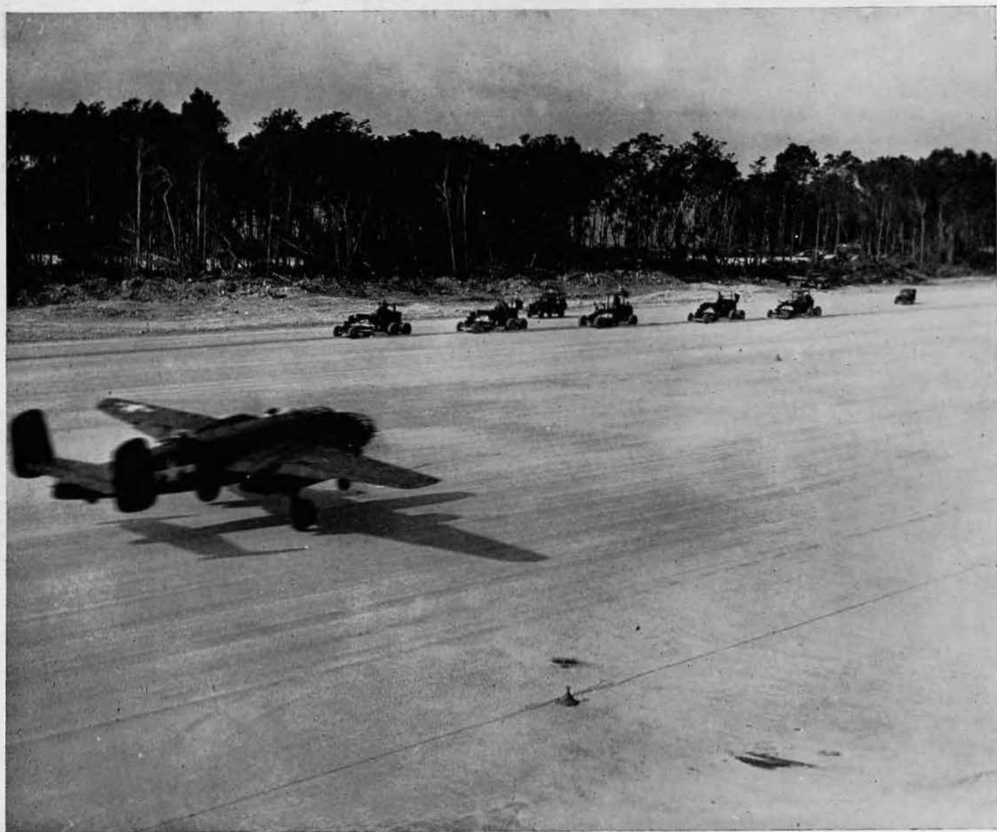
RAIDERS AND GRADERS. A B-25 takes off as part of a strike against last remaining Japs in the Solomons without interfering with a grading spread. It was usually necessary to clear runway when a mission was taking
