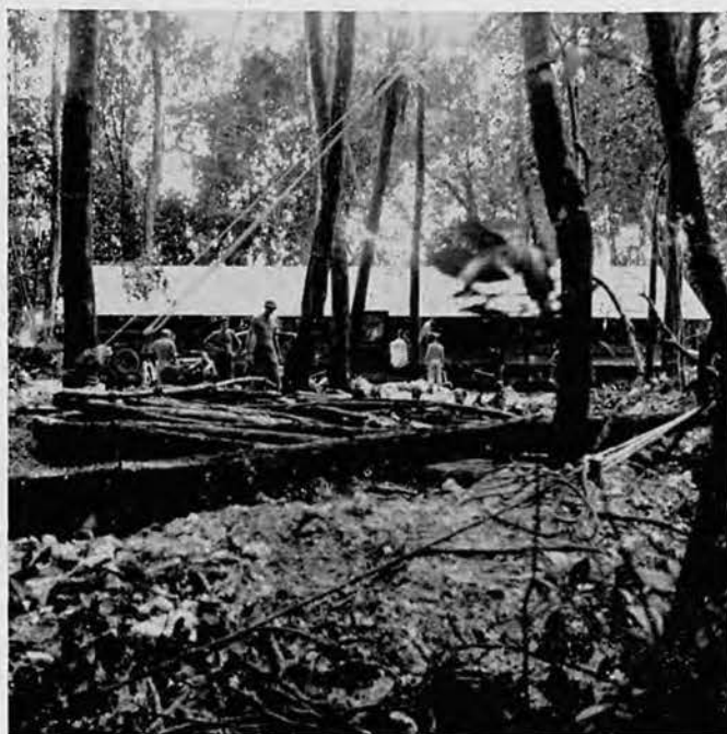
SICK BAY FOXHOLE. Chief William Martin and crew work hard constructing huge foxhole for 87th Sick Bay. The shelter accommodated 30 patients and was equipped with an emergency generator for use during alerts or when main power was not available.
