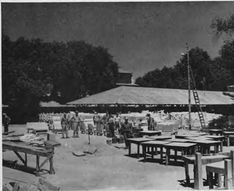
SETTING UP HOUSE. Prefabricated tables and really comfortable chairs were thrown together quickly once the basic construction was completed. Later painted in brilliant hues, the enlisted man's center had the rich carnival atmosphere of a gay beach resort.
