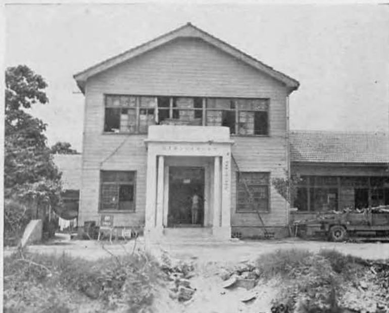
THROUGH THESE PORTALS pass American wounded from front line areas. This former Japanese military academy at Nago now houses the 87th Field Hospital. This structure was left virtually intact by invasion forces sweeping north.
