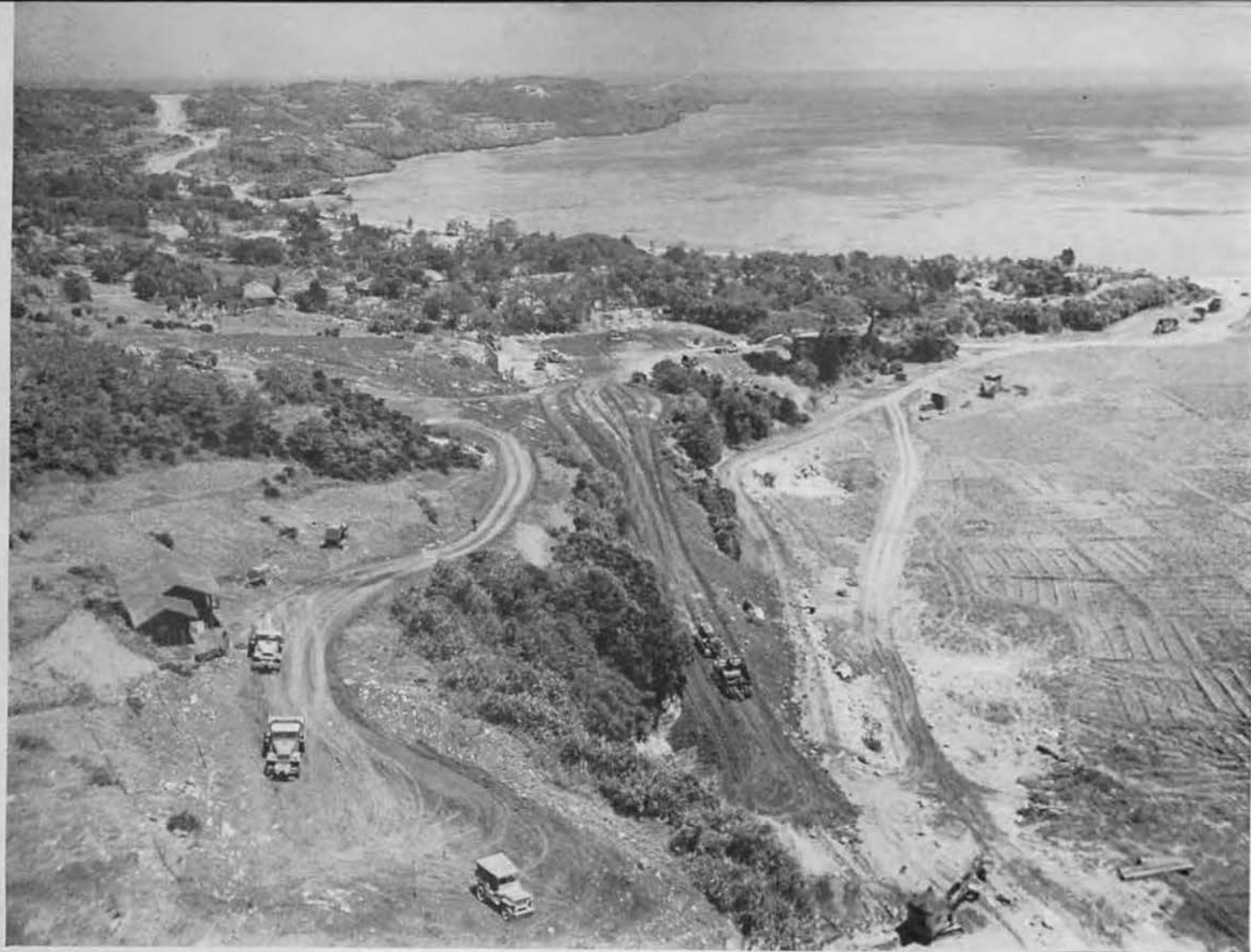
NAGAHAMA HARBOR (right center) is photographed from Face 1, near top of limestone mountain (see page 295). Taken before crusher assembly was installed, this shot shows site selected for rock crusher approximately in center of picture. Village of Nagahama spreads along waterfront of
