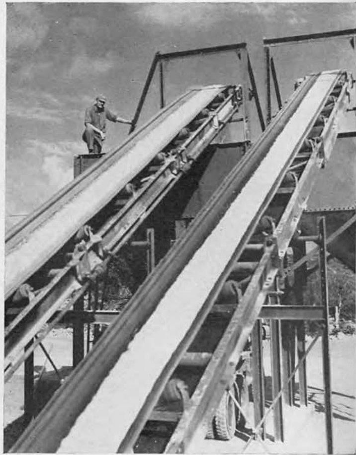
UP AND OVER. Ensign Frank Cizek observes flow of crushed stone along the conveyor belts into the gravity operated storage bins. The finished product varies in size up to 3/4-inch.
