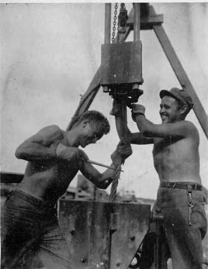
GENERAL RIGGING LOFT handled all assignments not pertaining to transportation equipment. Fred ("Buttercup") Haas (left) bellies his nickname as he executes a neat splice on a heavy cable. Tutor John ("Pinky") Doyle smiles down proudly upon his protegee.
