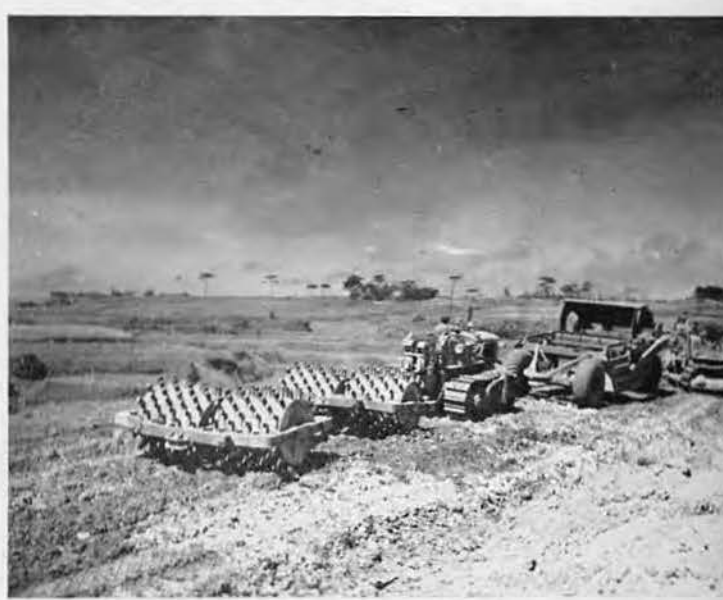
AT LAST. Actual work on Bolo Field commences on 19 June after many false starts and the 87th's last direct contribution toward winning the war is under way. Here, sheepfoot roller compacts fill behind 12-yard pan.
