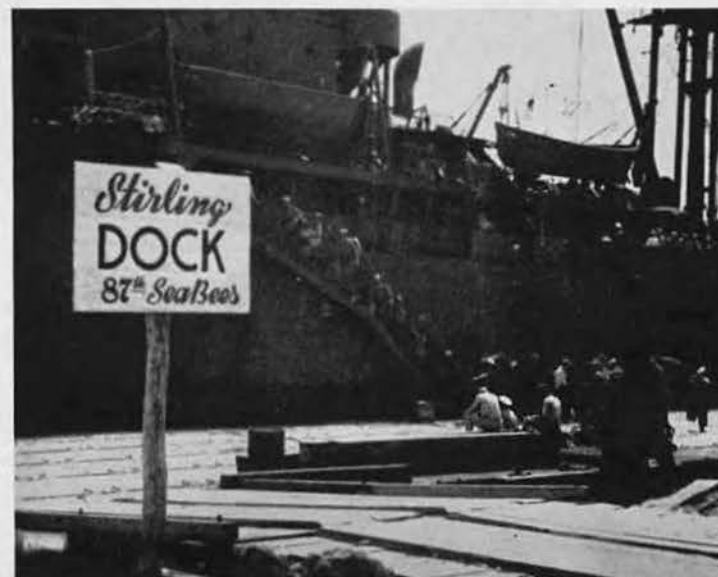
AND STILL THEY COME. Three CPOs sweat it out (seated on piling, right foreground) as endless lines continue up accommodation ladder. While the 87th builders are still given credit for Stirling Dock, gone forever is the famed sign, "What's Up, Dock?"
