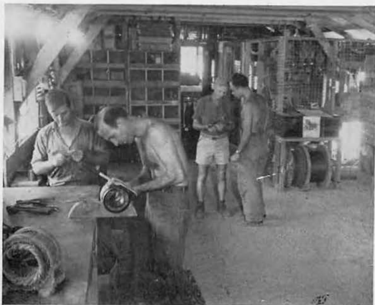
ELECTRIC SHOP handled repairs, rewinding and supplies. James Cheke and Bob Loden catch up bench work while Lieut. Davis explains defective coil to James Hockersmith. Here, these three were electrician's mates, first class; all eventually made CEM.
