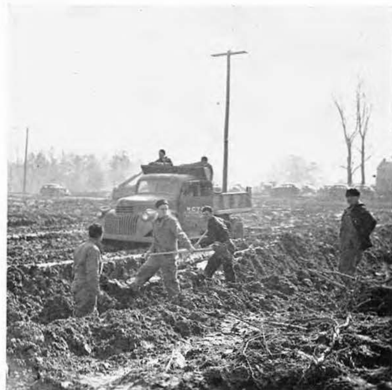
MUD ALL THE WAY UP was a depressingly familiar scene around Peary throughout boot days. They were building the sprawling camp when the boots arrived in February and it was still mushrooming when the 87th left in April.
