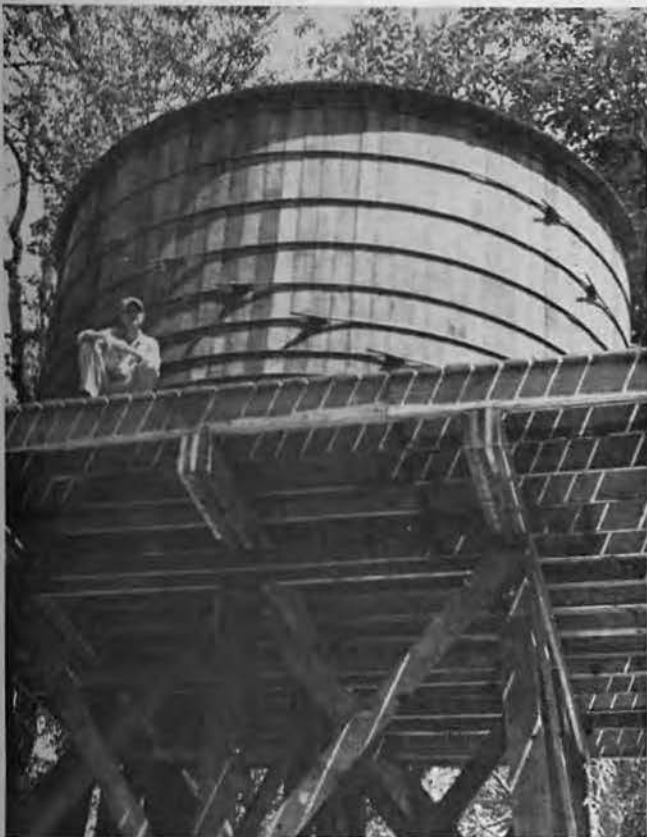
WATER TOWER. Towering virtually as high as the tallest surrounding jungle monarch, this imposing water tower supplies the pressure for the entire Camp Ostman water system. Perched high on the supporting platform, Lieut. William C. Reilly looks his project over.
